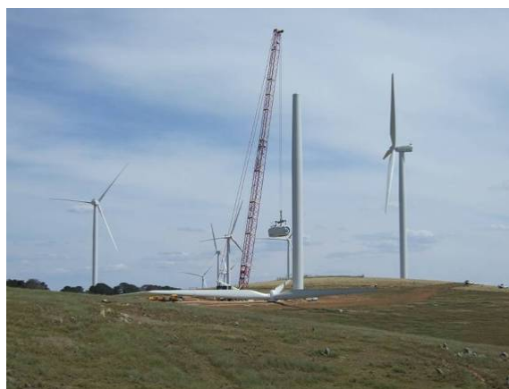
Plate 3.13 – Raising nacelle to install on tower as part of turbine erection.
