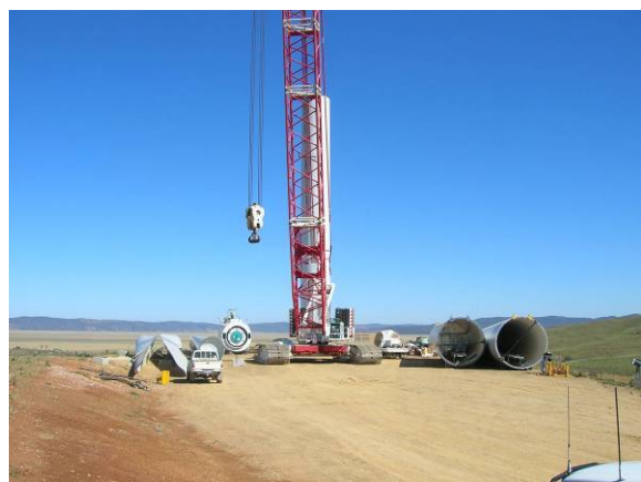
Plate 3.12 – Turbine components and crane on hardstand prior to turbine erection phase
