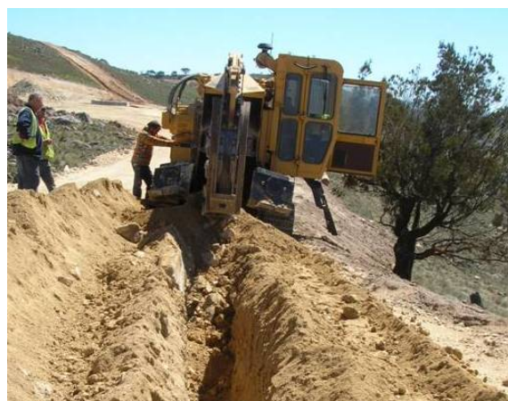
Plate 3.3 – Cable trench being excavated
