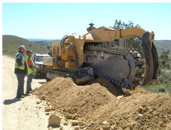
Plate 3.2 – Typical trenching machine
