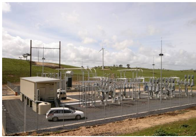
Plate 3.5 – View of 132 kV Substation for the 46 turbine Lake Bonney Stage 1 Wind Farm
