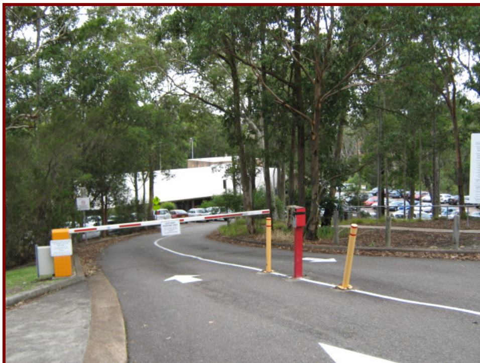
Photograph 2: View of existing entrance, known as Guntree Close, to the former staff amenities building and car park.
