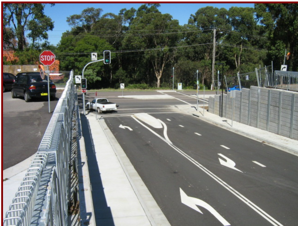
Photograph 14: View of intersection of Jacaranda Drive and Croudace Street. Jacaranda Drive is a relatively new access road, constructed in 2007.
