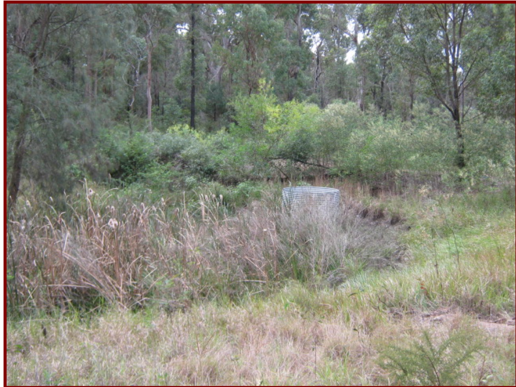
Photograph 12: View of the existing detention basin to the east of the development site, which has the capacity to accommodate increased detention requirements.
