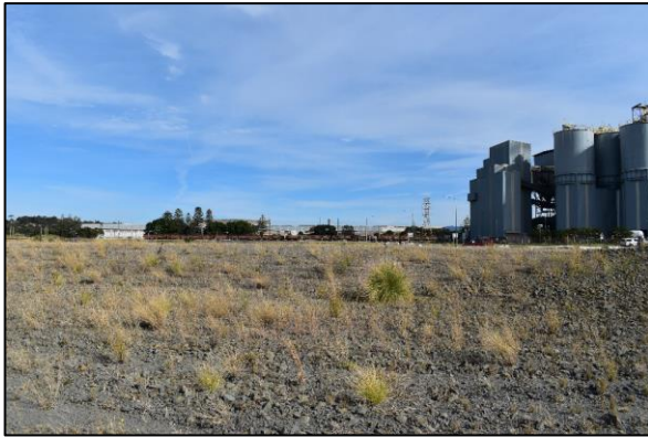
Figure 20: View southwest SEPP Item 1 (behind pines and other trees) from within the proposed works area
