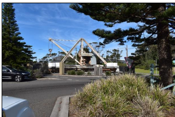
Figure 28: View of the Mobile Block Setting Steam Crane and towards heritage items and study area
