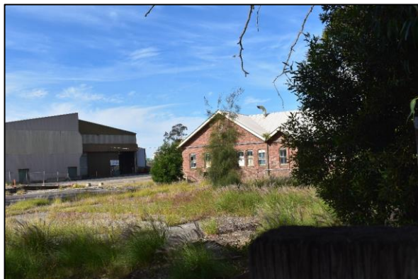
Figure 30: View north from SEPP item 2 (Brick structure) towards study area proposed works (obscured behind shed in background)
