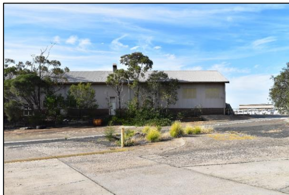
Figure 31: Views from SEPP items 2 (Brick structure) towards study area (behind shed in background)
