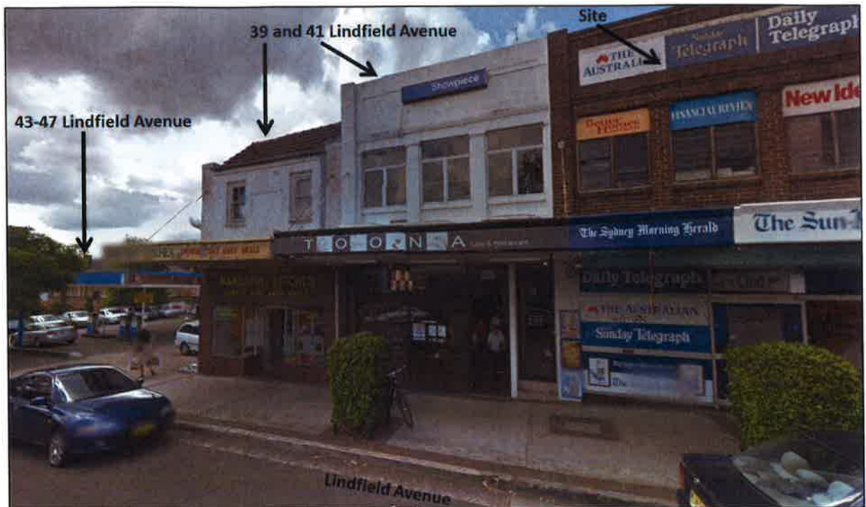
Figure 2: View looking north from Lindfield Avenue showing site (right) site 39-41 Lindfield Avenue (middle) and 43-47 Lindfield Avenue (left)
