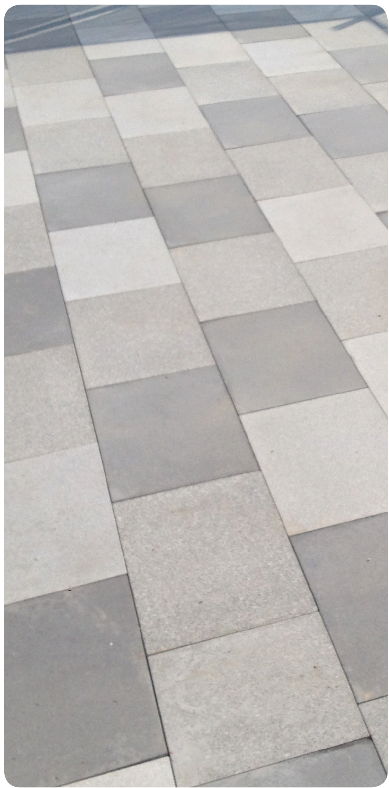
Large Format Urbanstone Paver at Gordon Interchange Depth 60mm Size 600x400/400x400/400x200mm
