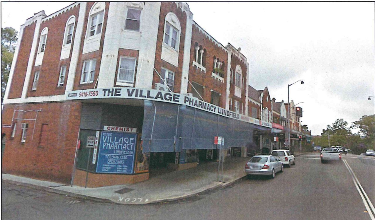
Figure 6: View looking south from the intersection of Lindfield Avenue and Kochia Lane of heritage listed building at 1-21 Lindfield Avenue
