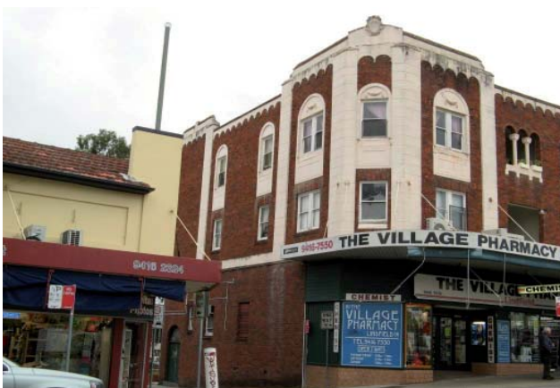
Figure 2.12 View of the existing building at 23 Lindfield Avenue, showing its relationship to the listed building at 1-21 Lindfield Avenue, separated by Kochia Lane
