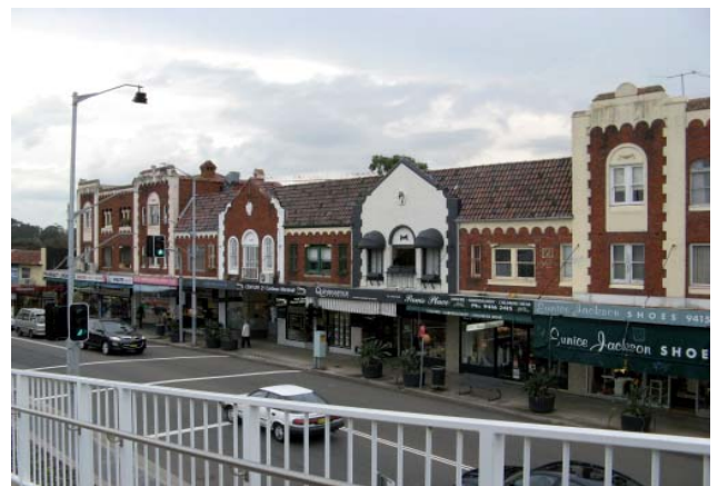
Figure 2.11 View of the listed building at 1-21 Lindfield Avenue, looking north from the vicinity of the railway station pedestrian ramp
