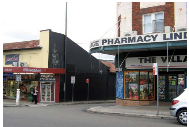
Figure 2.13 View of the existing building at 23 Lindfield Avenue, showing its relationship to the listed building at 1-21 Lindfield Avenue, separated by Kochia Lane
