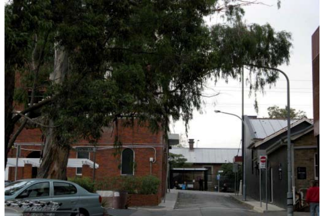
Figure 2.15 View of the existing building at 23 Lindfield Avenue (on the right), showing its relationship to the listed building at 1-21 Lindfield Avenue (on the left), separated by Kochia Lane. Lindfield Railway Station is seen at the rear of the image between the two buildings
