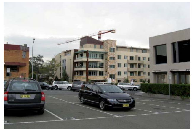
Figure 2.7 Recent development at the corner of Kochia and Havilah Lanes and the commercial building adjoining the south east corner of the subject site
