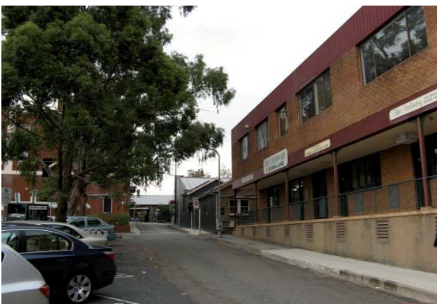
Figure 2.6 Looking west along Kochia Lane showing the interface between the heritage listed building (on the left) and the subject site, with Lindfield Station seen in the background, at the end of the lane
