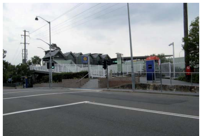
Figure 2.19 View to the northern end of Lindfield Railway Station from the vicinity of the subject site
