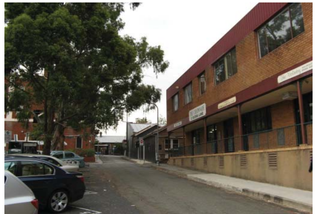
Figure 2.9 Looking west along Kochia Lane showing the interface between the heritage listed building (on the left) and the subject site
