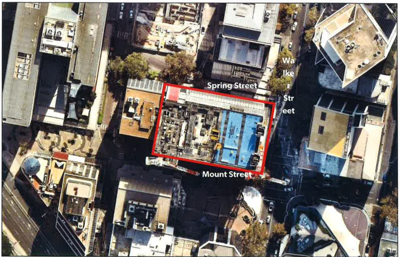
Figure 2: Aerial photo showing construction on the site (Source: Nearmap)
