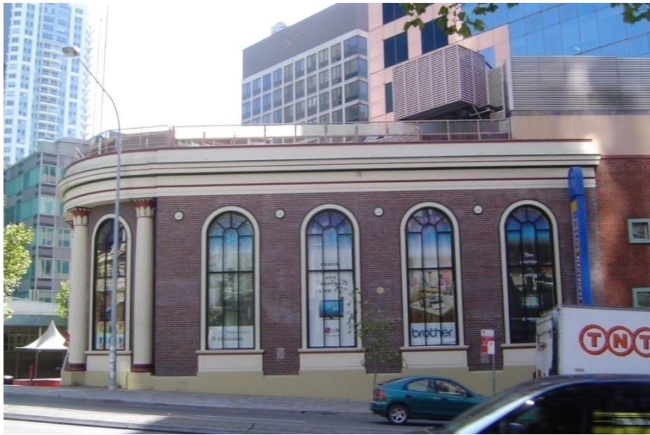
Figure 21: The Bank of NSW (Former) Miller Street View from the West
