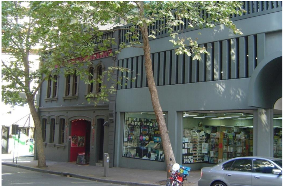
Figure 9: Former North Sydney Fire Station, View from north on Walker Street
