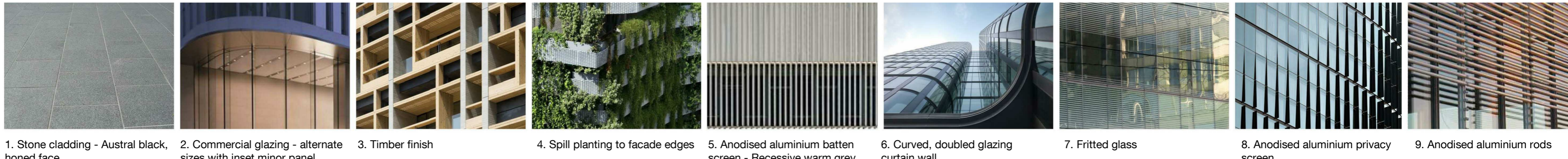
1. Stone cladding - Austral black, 2. Commercial glazing - alternate sizes with inset minor panel, 3. Timber finish honed face, 4. Spill planting to facade edges, 5. Anodised aluminium batten screen - Recessive warm grey, 6. Curved, doubled glazing curtain wall, 7. Fritted glass, 8. Anodised aluminium privacy screen, 9. Anodised aluminium rods
