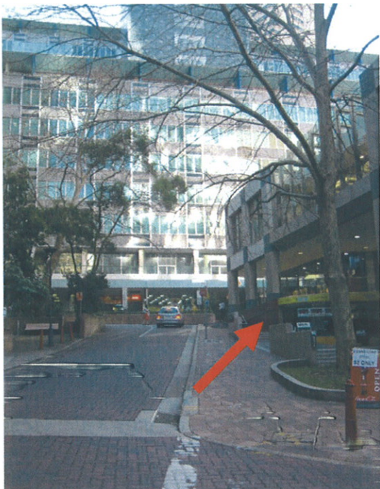
Photo 1 – Looking west along Spring Street
