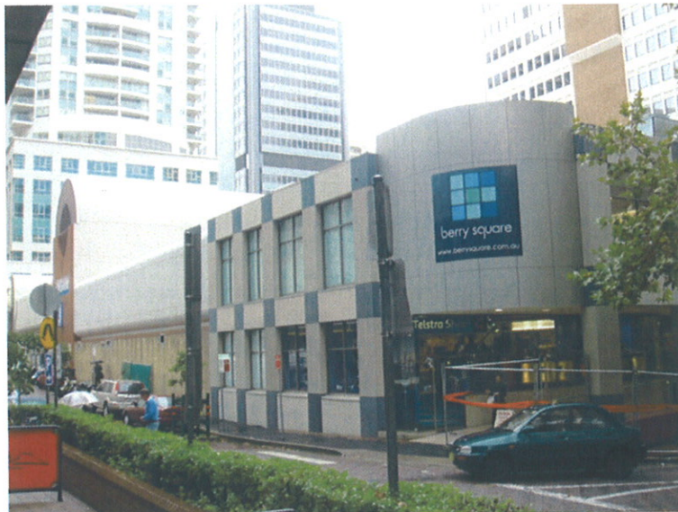
Photo 3 - Looking north-east across intersection of Spring Street and Denison Street
