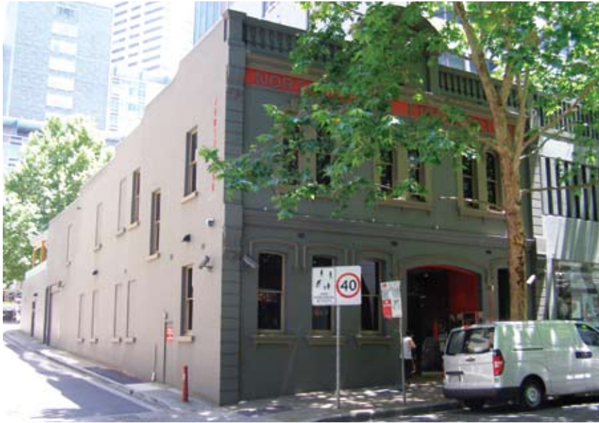
Figure 18 – The heritage listed Firehouse Hotel (86 Walker Street)
