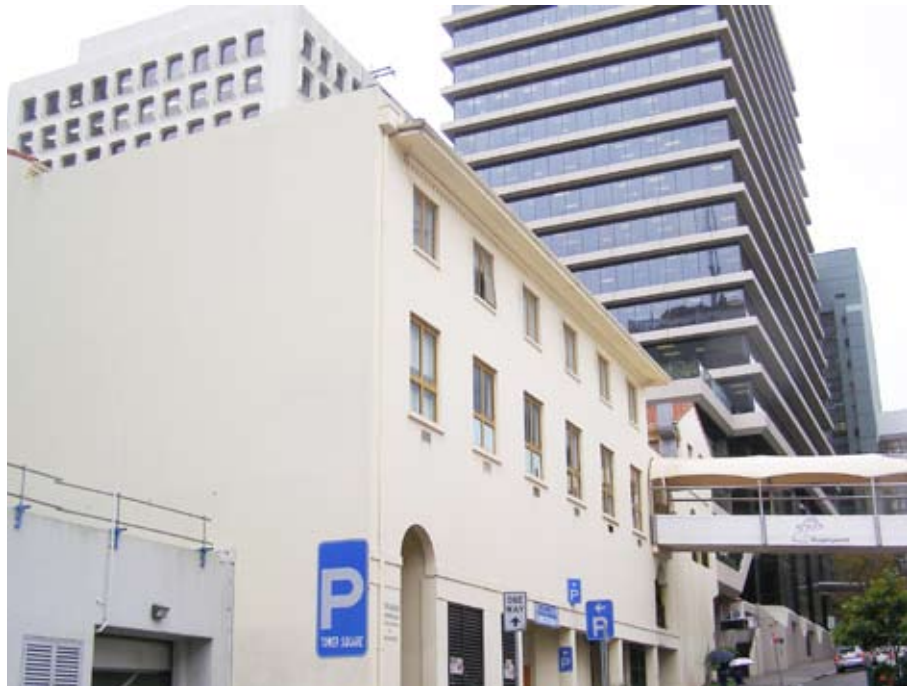
Figure 16 – Tower Square Development (Miller Street)
