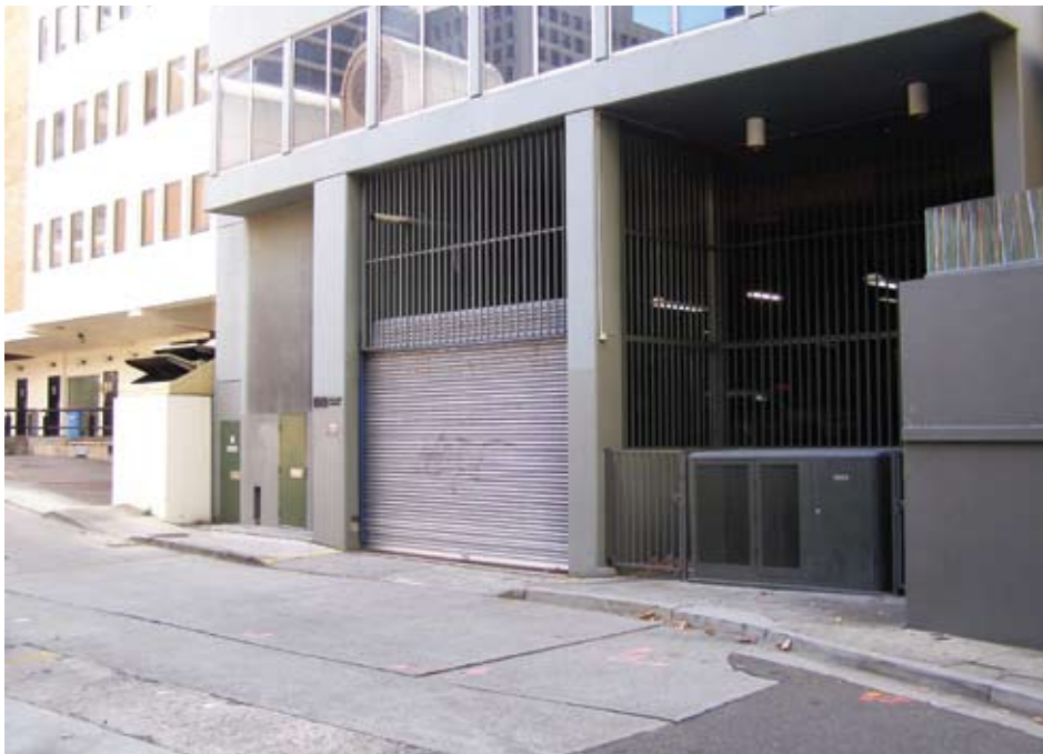
Figure 10 – Entrances to 88 Walker Street basement carpark
