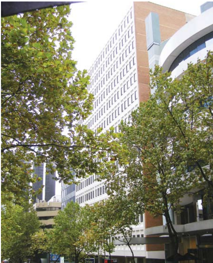
Figure 19 – Adjacent commercial building to the north (100 Walker Street)
