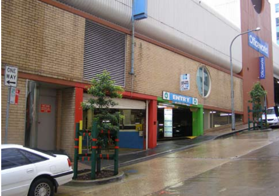
Figure 9 – Entrance to Berry Square Retail (77 Berry Street) basement carparking and loading dock
