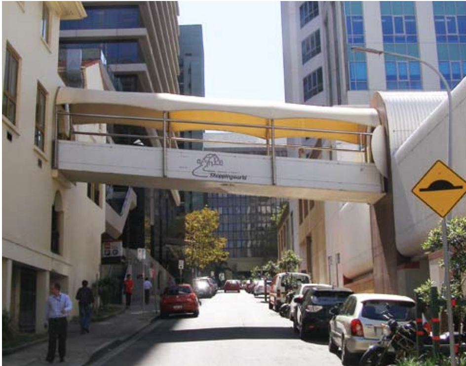
Figure 6 – Pedestrian bridge linking 77 Berry Street with Tower Square
