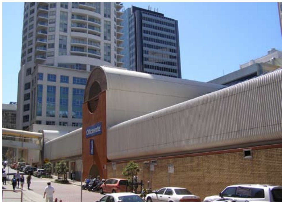
Figure 5 – Berry Square Retail as viewed from Denison Street
