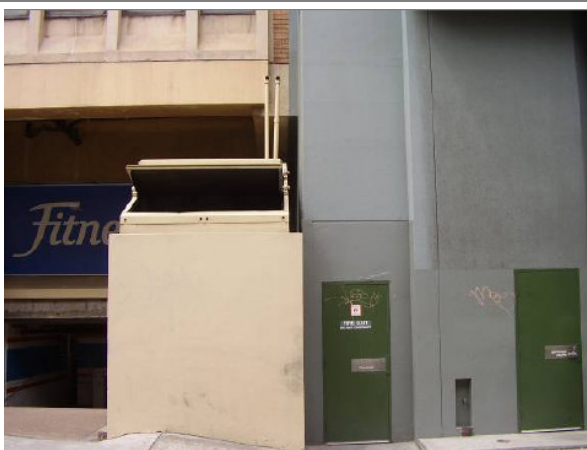
Figure 17 - Vent lines of potential UST at adjacent property to the north
