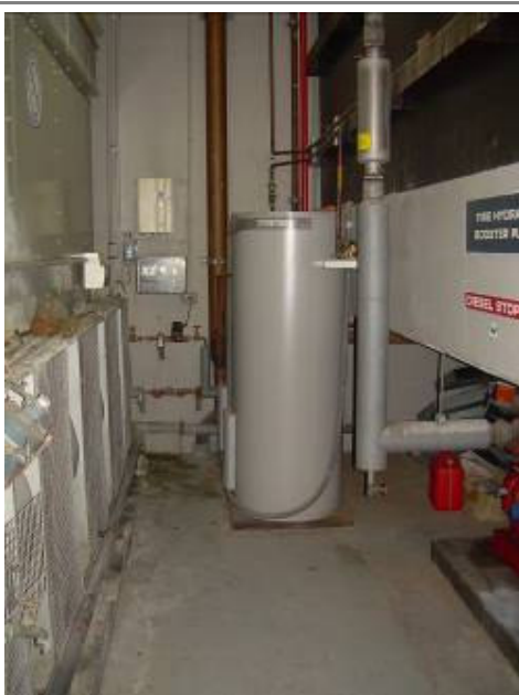
Figure 7 - Rooftop fire hydrant booster pump
