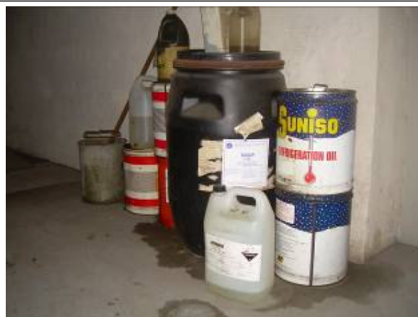
Figure 10 - Rooftop miscellaneous chemicals stored beneath the Lift Motor Room
