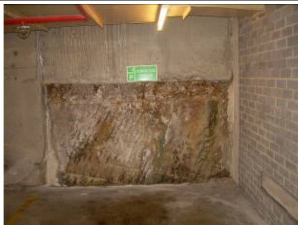
Figure 20 - Car park cut into bedrock
