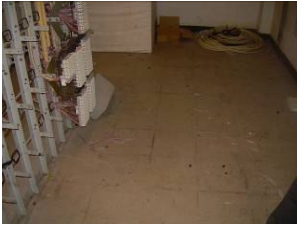
Figure 21 - Vinyl tiles in the MDF room.
