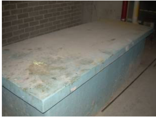
Figure 22 - Decommissioned grease trap at the northern end of the car park.
