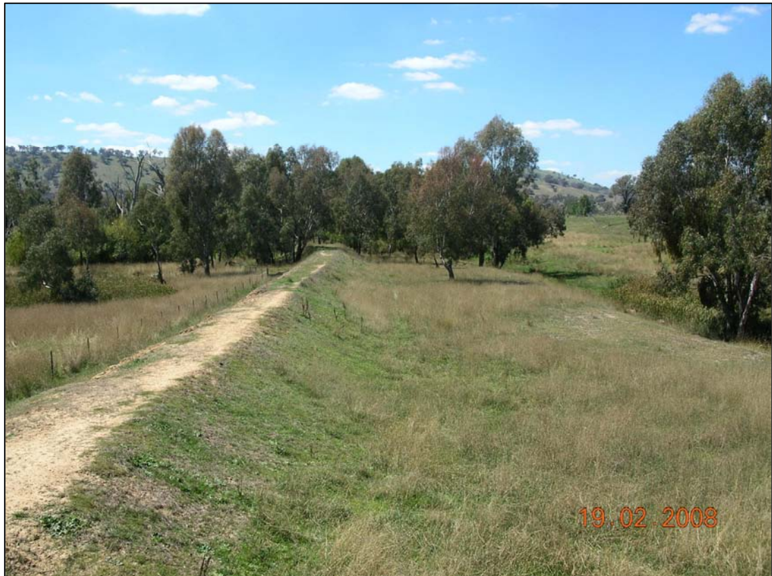
Mountain Creek at Fairbain Road Bridge – Looking upstream at levee
