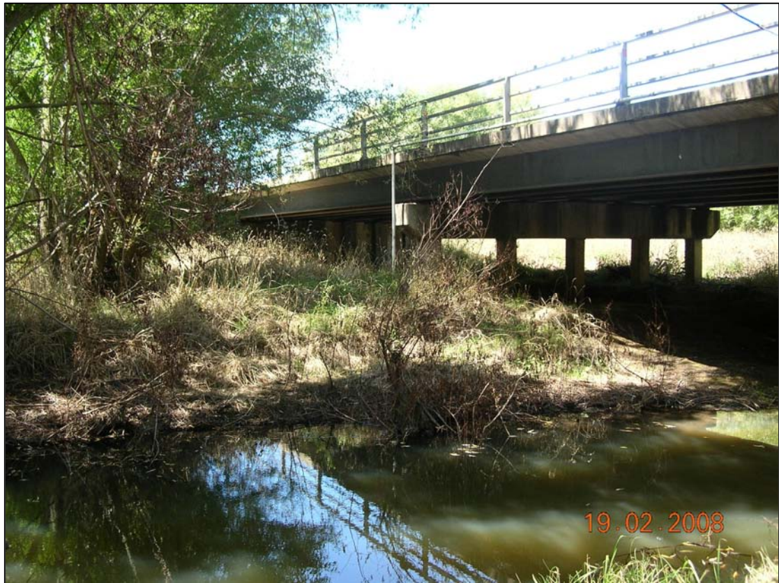
Mountain Creek – Existing Hume Highway Bridge crossing, looking upstream
