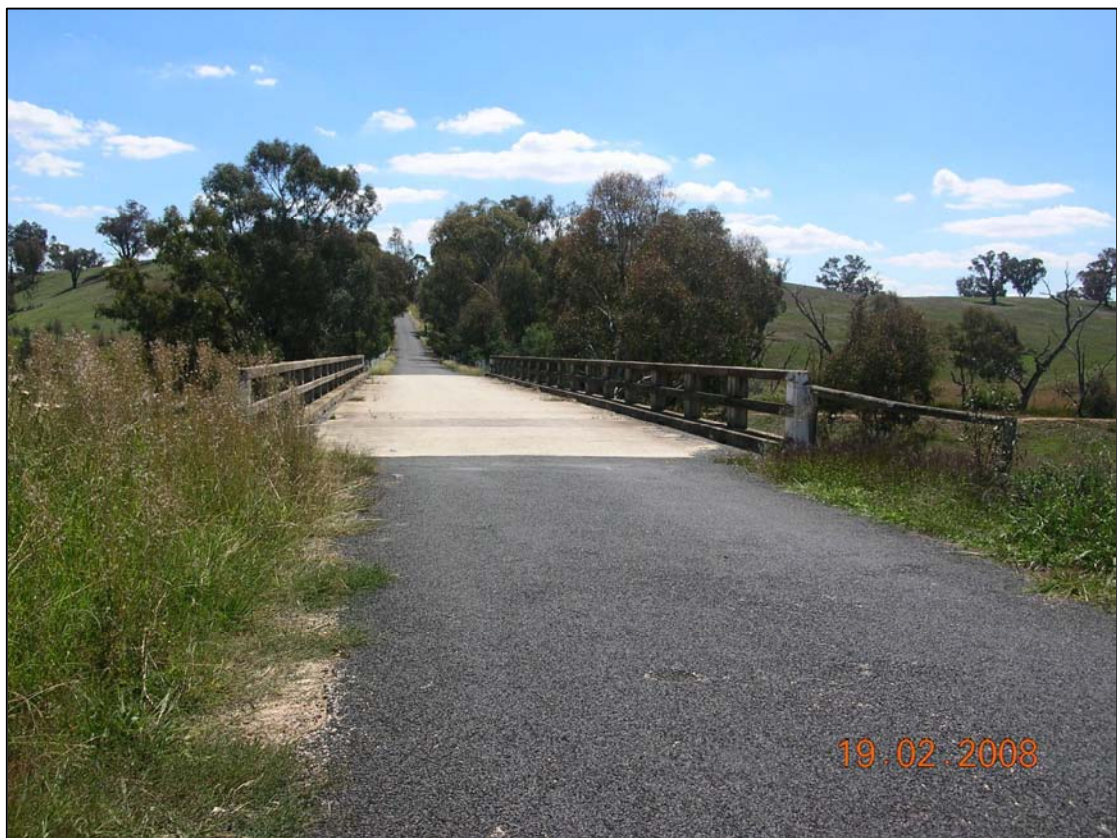
Fairbain Road – Bridge crossing of Mountain Creek, looking west
