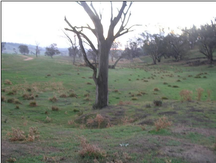
Photograph 3-9 Dam D3 – downstream
