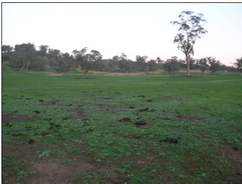
Photograph 3-11 Dam D5 – upstream
