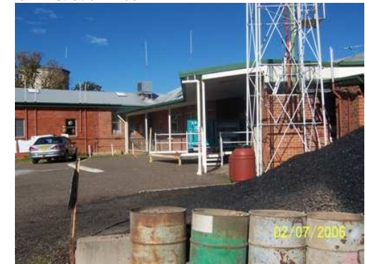
Plate 4.27: Hospital additions are obvious to the entire building.
