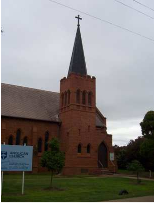
Plate 3.11: Anglican Church on Stratford Street.
