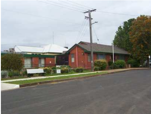
Plate 3.1: View of the Administration Block
