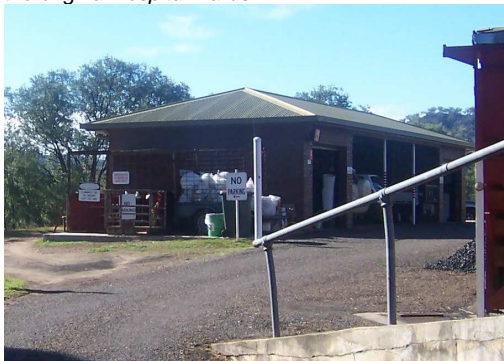
Plate 4.26: Modern Workshop building at the rear of the site.
