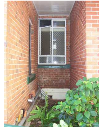
Plate 4.10: a metal framed window installed as part of an upgrade.
