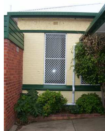
Plate 4.7: Painted original hospital brick walls.
