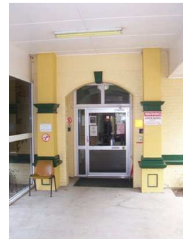
Plate 4.16: View of the original hospital entrance archway noting the simple key stone, which appears smaller than the one in the photos of the original building.
