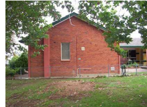
Plate 4.25: The north-eastern end of the Administration Block.
