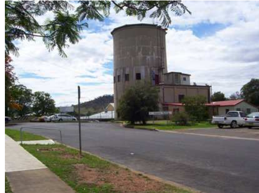
Plate 3.2: View of the council water tower opposite.
