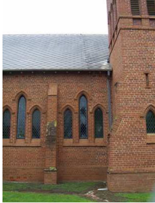
Plate 3.12: Anglican Church on Stratford Street.
