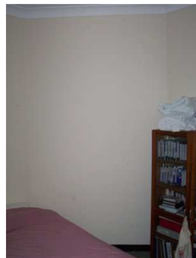
Plate 4.14: Corner fireplace removed from wall.
