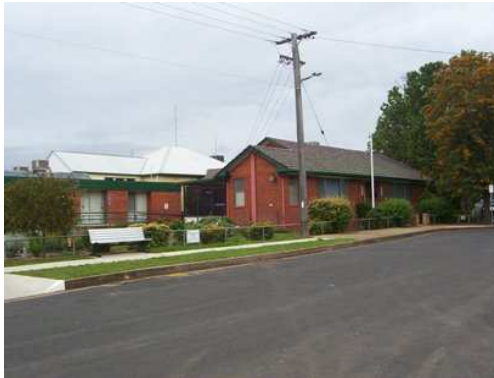
Plate 4.3: The 1962 brick Administration building and 1977 brick Ward additions.
