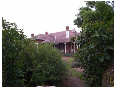
Plate 3.12: Entry to house on Stratford Street.
