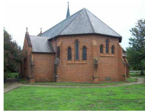
Plate 3.10: Anglican Church on Stratford Street.
