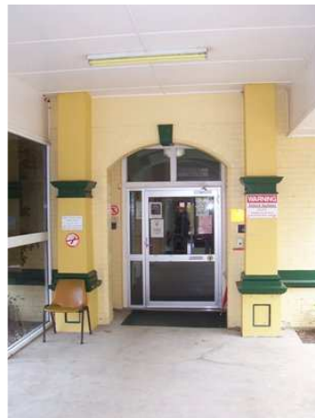
Plate 4.6: Painted original hospital brick walls.
