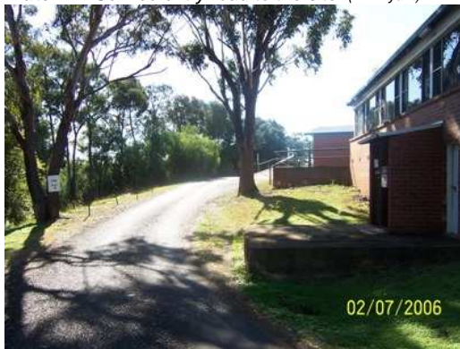
Plate 7.3: Internal road north of the hospital. (W. Bryant)
