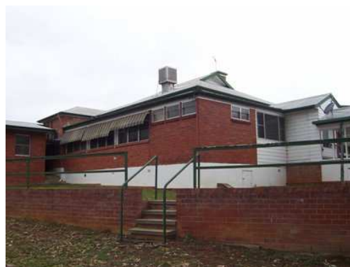
Plate 4.21: The original 1909 Nurses Quarters building with enclosed verandahs.
