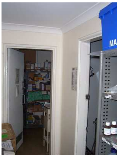
Plate 4.13: Early joinery to doors of the 1916 Operating Theatre.
