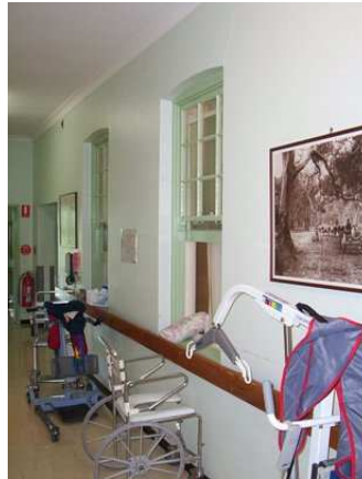
Plate 4.9: An external wall & timber double hung window forms part of a corridor.
