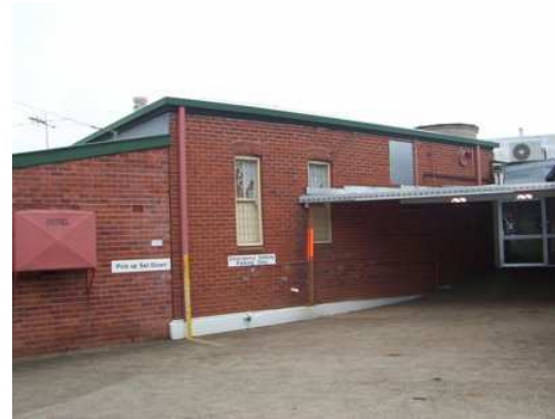
Plate 4.4: The 1916 face brick Hill Operating Theatre additions to the original hospital buildings.
