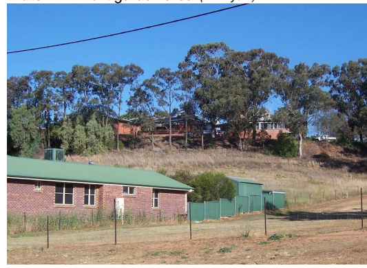
Plate 7.4: Hospital viewed from the north. (W. Bryant)
