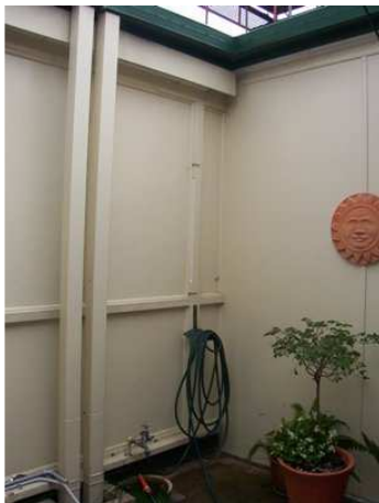
Plate 4.5: The partition walls typical of the 1930's Parkes additions.
