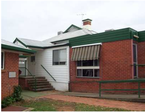
Plate 4.22: The original 1909 Nurses Quarters building with original chimney in good condition.
