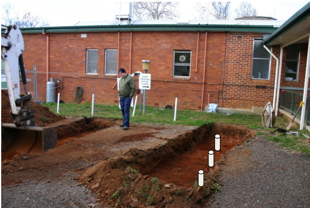
Figure 3.6 Test Trenches in progress. Carney (2009). White stumps indicate approximate post alignment (not height or shape).
