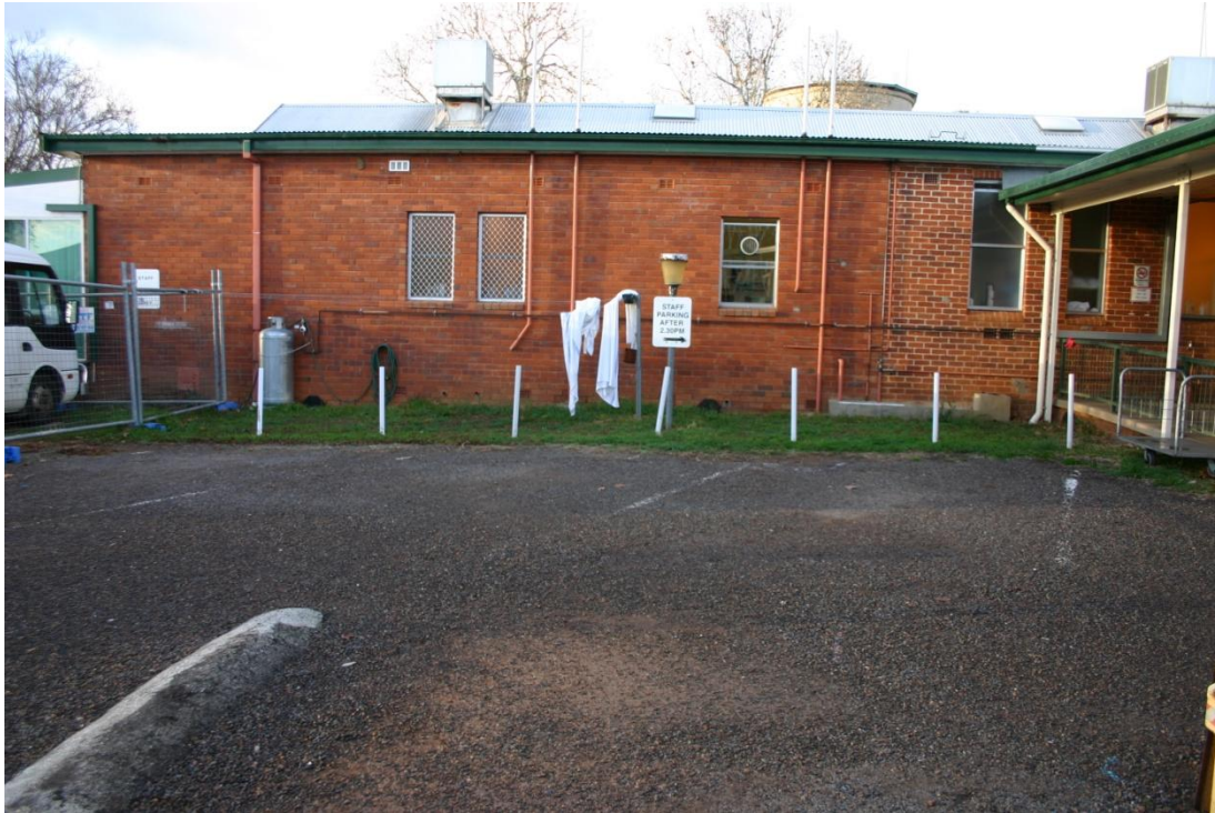
Figure 3.5 Test Trench Location Carney (2009).
