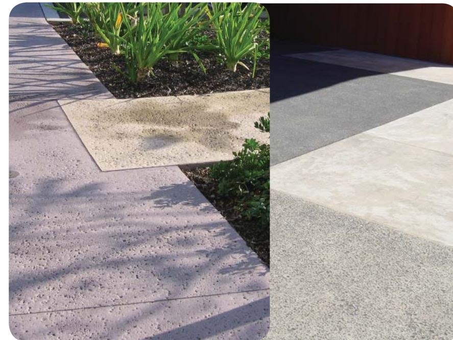
Coloured in-situ concrete paving
