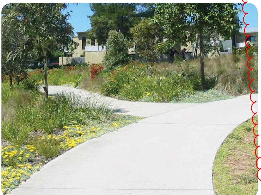
Coloured in-situ concrete pathway
