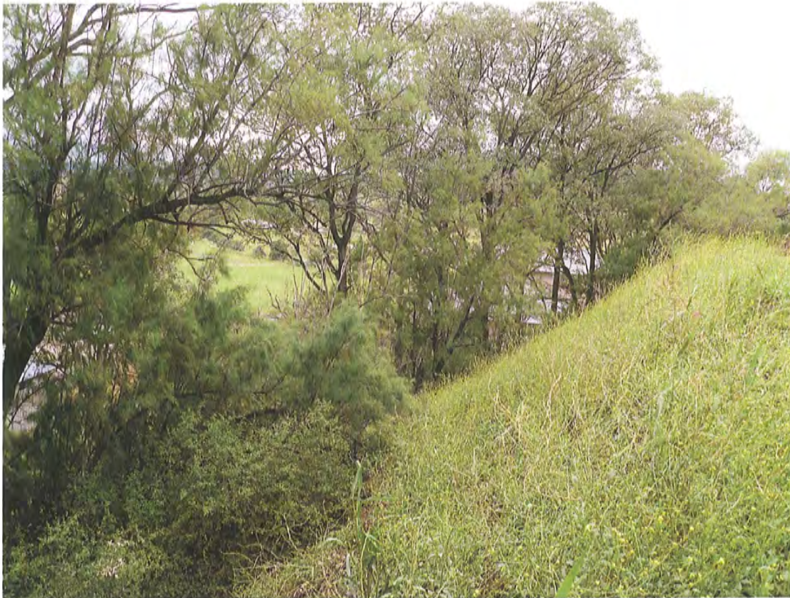
Plate 7: View of the filled batter, opposite the coal bin, looking east/north-east towards the workshop. Batter is overgrown with native grasses. The perimeter fence is tree-lined.
