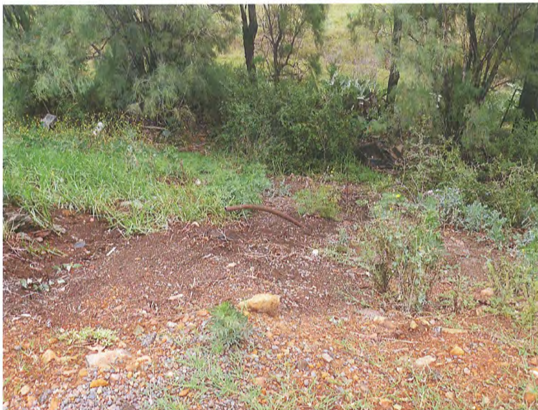
Plate 13: Close up of fill materials in the batter at the rear of the workshop.
