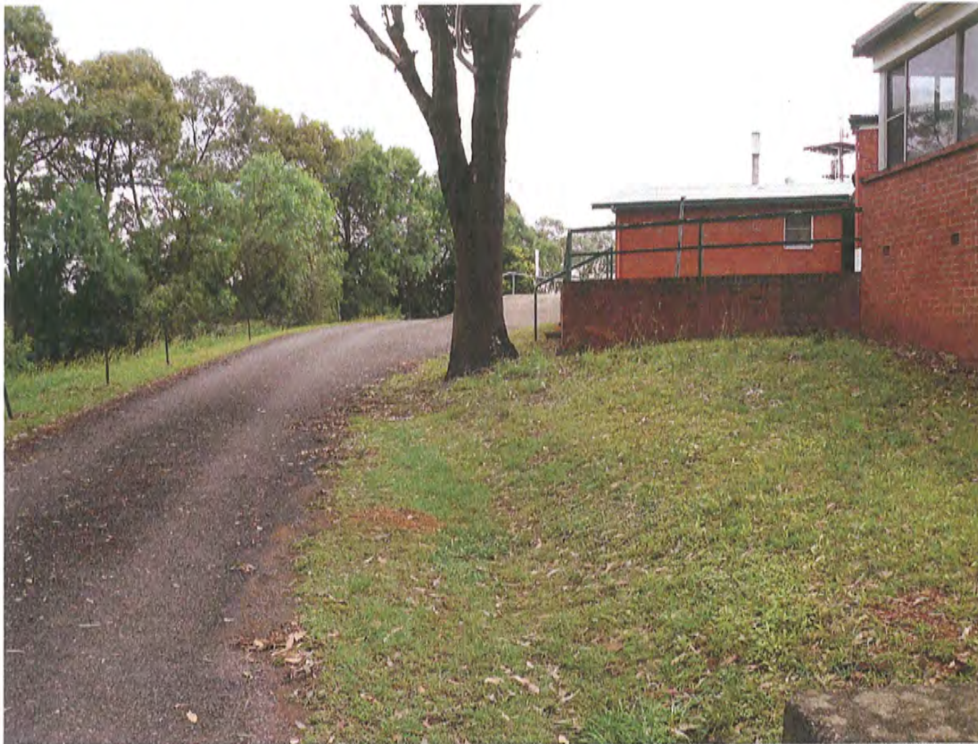
Plate 3: View of the access road, looking north-east from the rear of nurses quarters.
