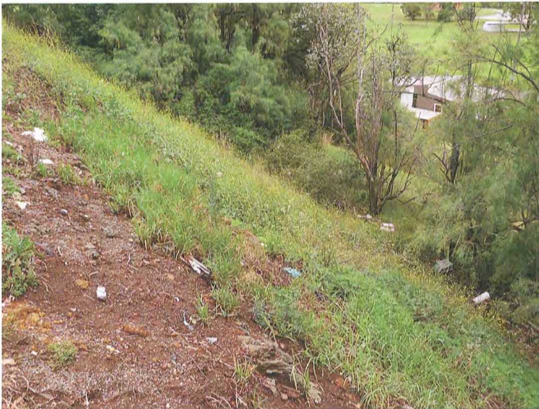
Plate 8: View of the fill batter at the rear of the workshop, looking north-west.
