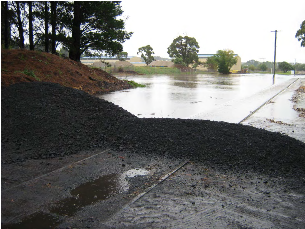
Figure 6 | Temporary bund across rail line
