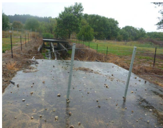
Plate 16: Survey Unit (1e) – View of a large concrete slab over wooden beams
