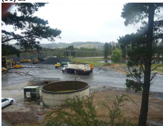
Plate 9: Survey Unit (1c) – View of coal loading and stock pile
