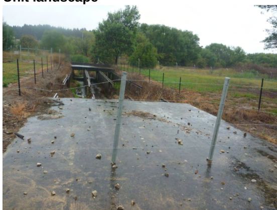
Plate 17: Survey Unit (1e) – View of a large concrete slab over wooden beams
