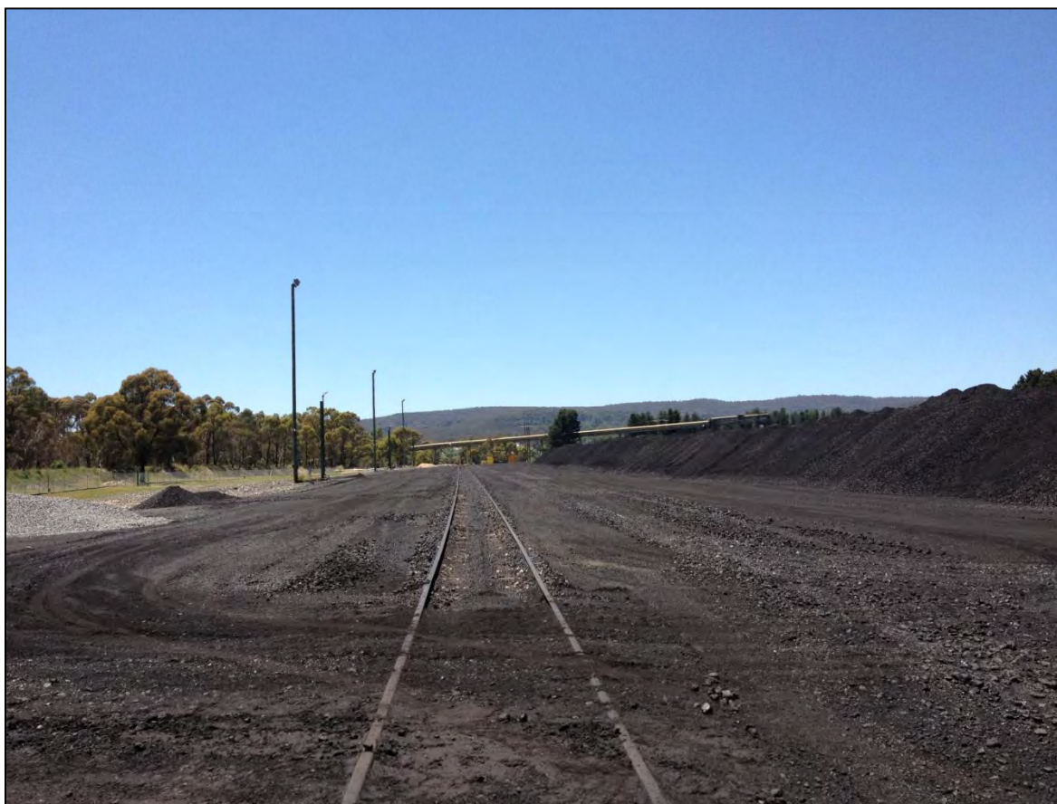
Plate 3-14: (Location 6) Lidsdale Rail Line (looking north)
