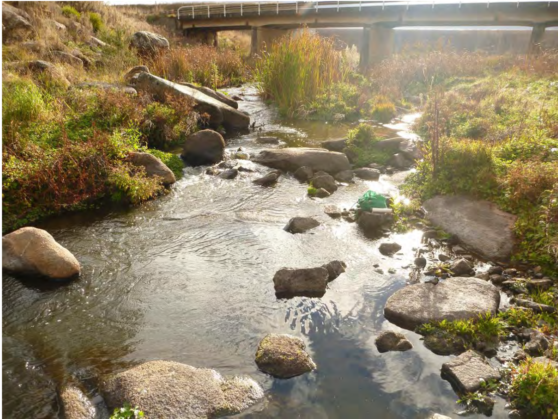
Plate 28: Looking upstream at CR6.
