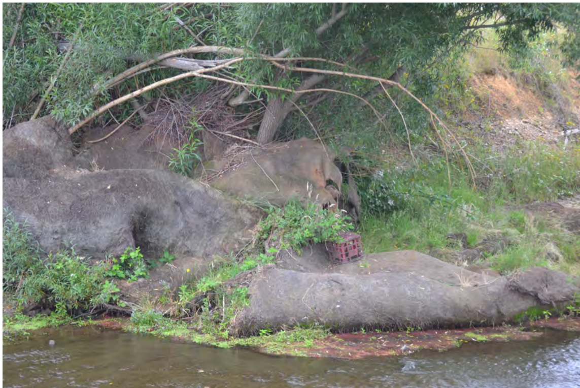
Figure 5 Photo of nick point in Pipers Flat Creek diversion channel where willows have established. Storm flows prior to the date of this photo (20 December 2011) had uprooted some of the willows and flow under the root mat has doubled the willow root mat over itself as indicated, partially clearing the creek obstructions at this point.
