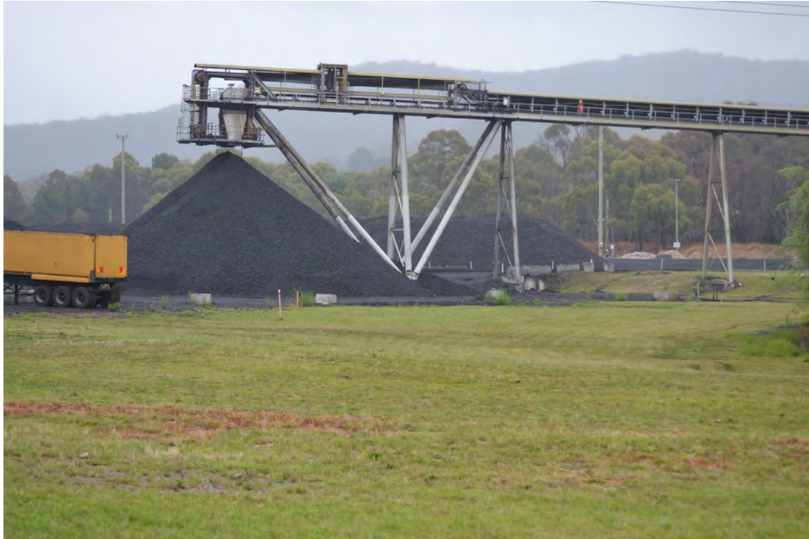
Lidsdale Siding Coal Conveyor
