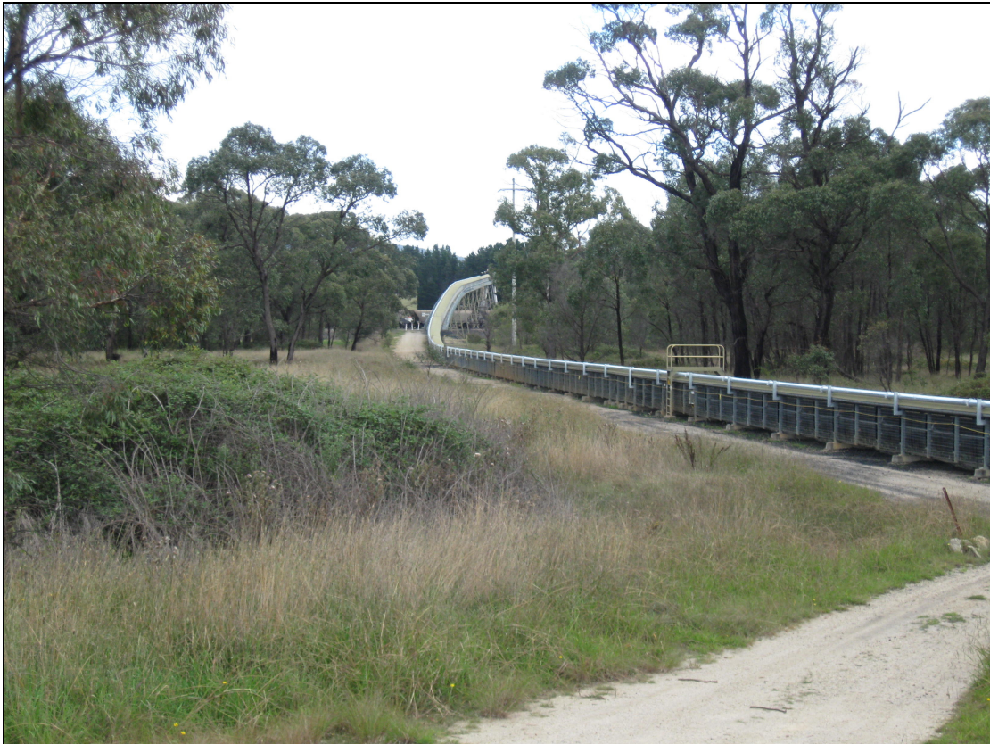
Plate 6: Overland Conveyor from Coal Services looking South from Brays Lane
