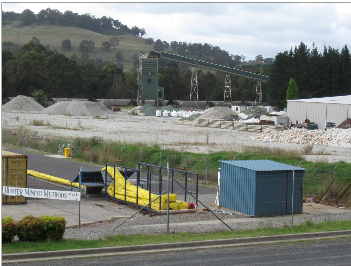
Plate 9: Montage of New Rail Loading Bin and Feed Conveyor
