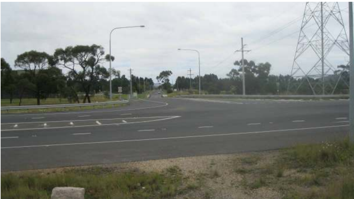
Plate #2 – Existing road intersection, Castlereagh Highway & Main Street, Wallerawang
