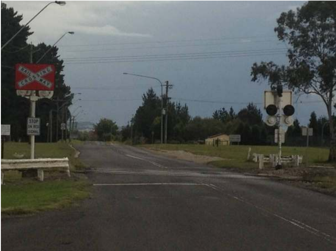
Plate #1 – Existing rail level crossing, Main Street, Wallerawang
