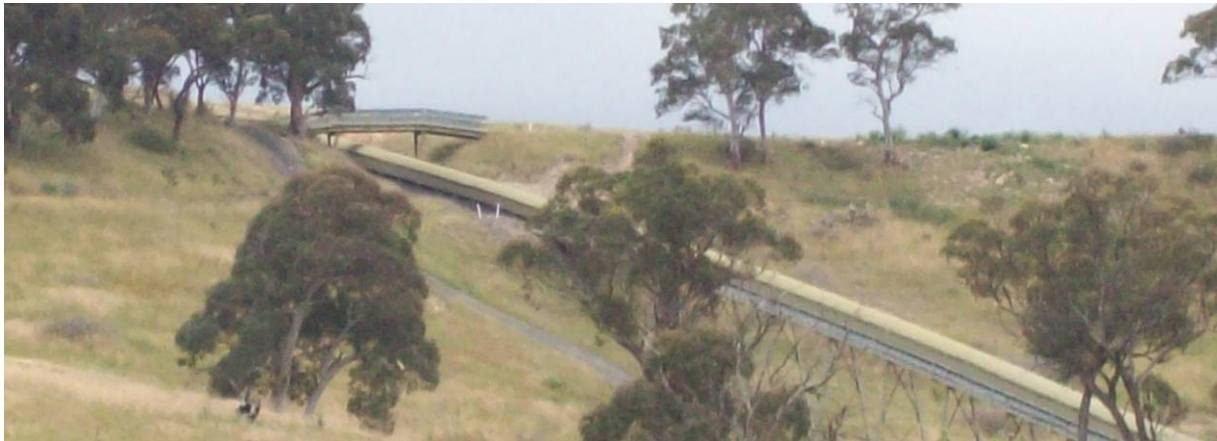
Overland conveyer, Duncan Street
