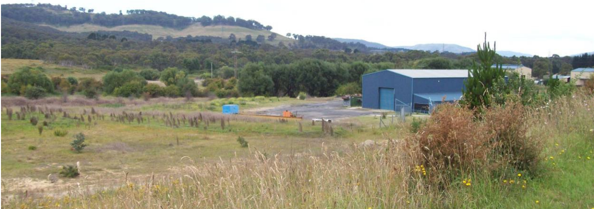
The existing rail siding has been effectively buffered by both natural vegetation and industry.
