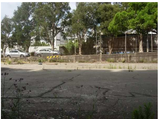
Figure 4.10. View to the east demonstrating the level of the site and the level of Pymont Street. Approximate location of bore hole 2.
