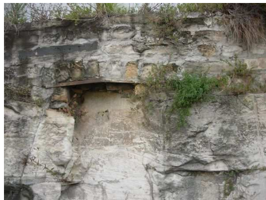
Figure 4.5. Overhanging retaining wall section supported by an iron lintel.
