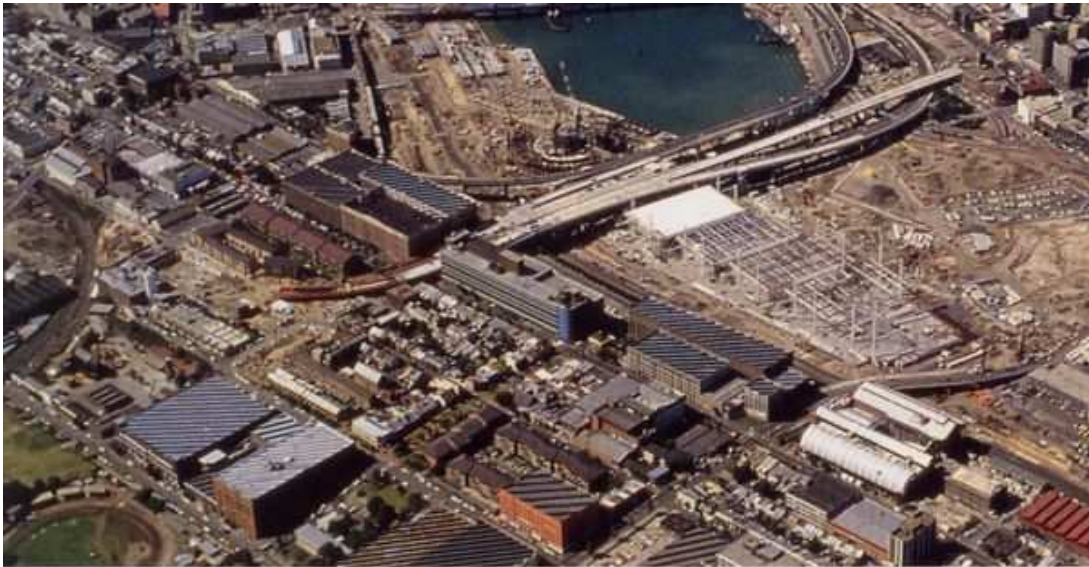
Figure 3.10. Aerial view of the redevelopment of Darling Harbour 1987. The Government Printers Office is in the centre of the image. The subject site is vacant (Photograph courtesy of SHFA).
