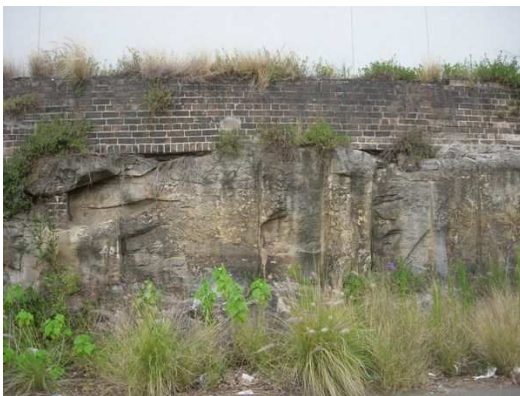
Figure 4.4. Vegetation growing along the rock face and retaining wall on the western perimeter of the site.
