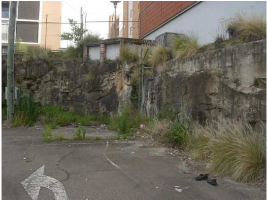
Figure 4.6. The south west corner of the site, view toward Quarry Street demonstrating the depth of exposed bedrock. Approximate location of bore hole 1.
