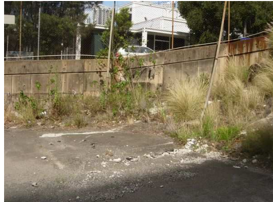
Figure 4.7. The south east corner of the site showing the sloping grade of Quarry Street (on the right) down to Pymont Street.
