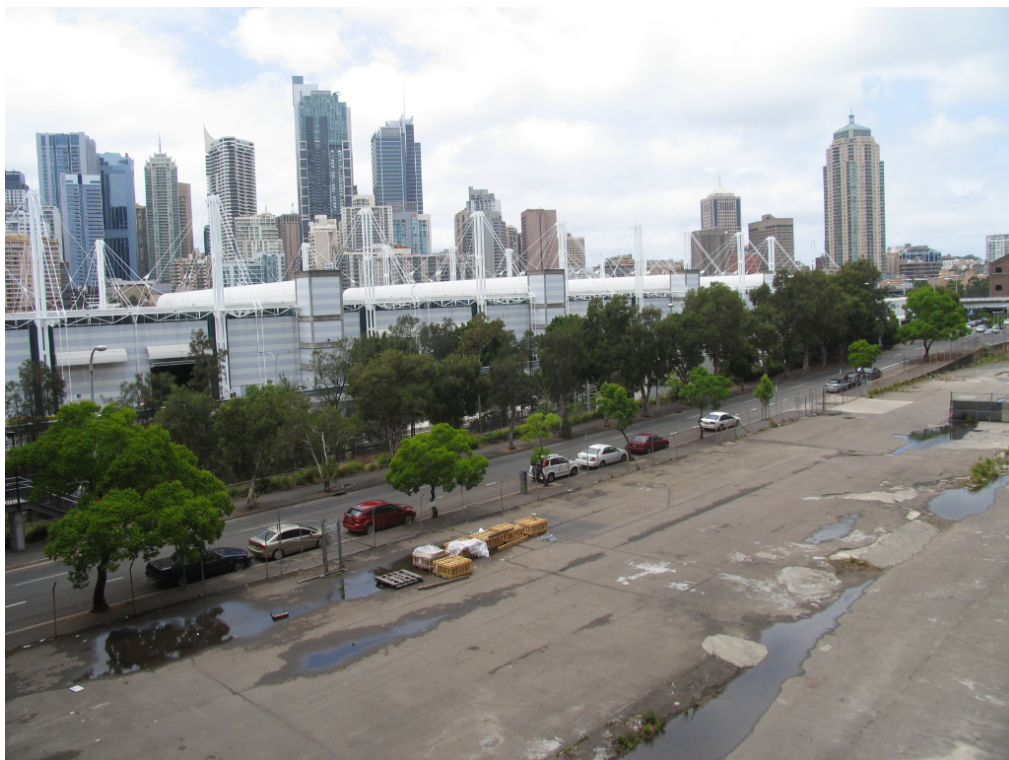
Photo 6 – Looking south-east over site towards Darling Harbour and the City skyline
