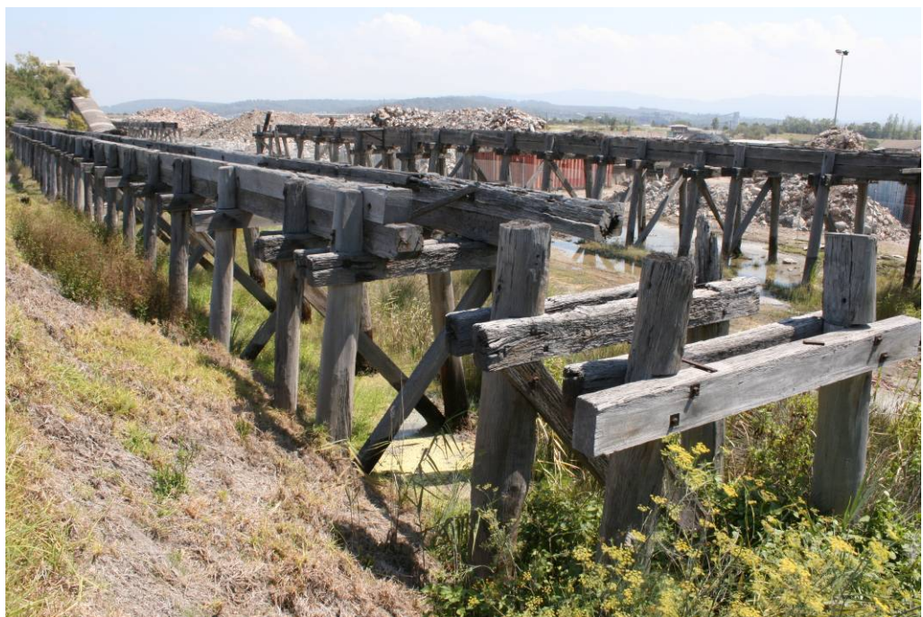
Photograph A.24 Wooden A frame gantry on site
