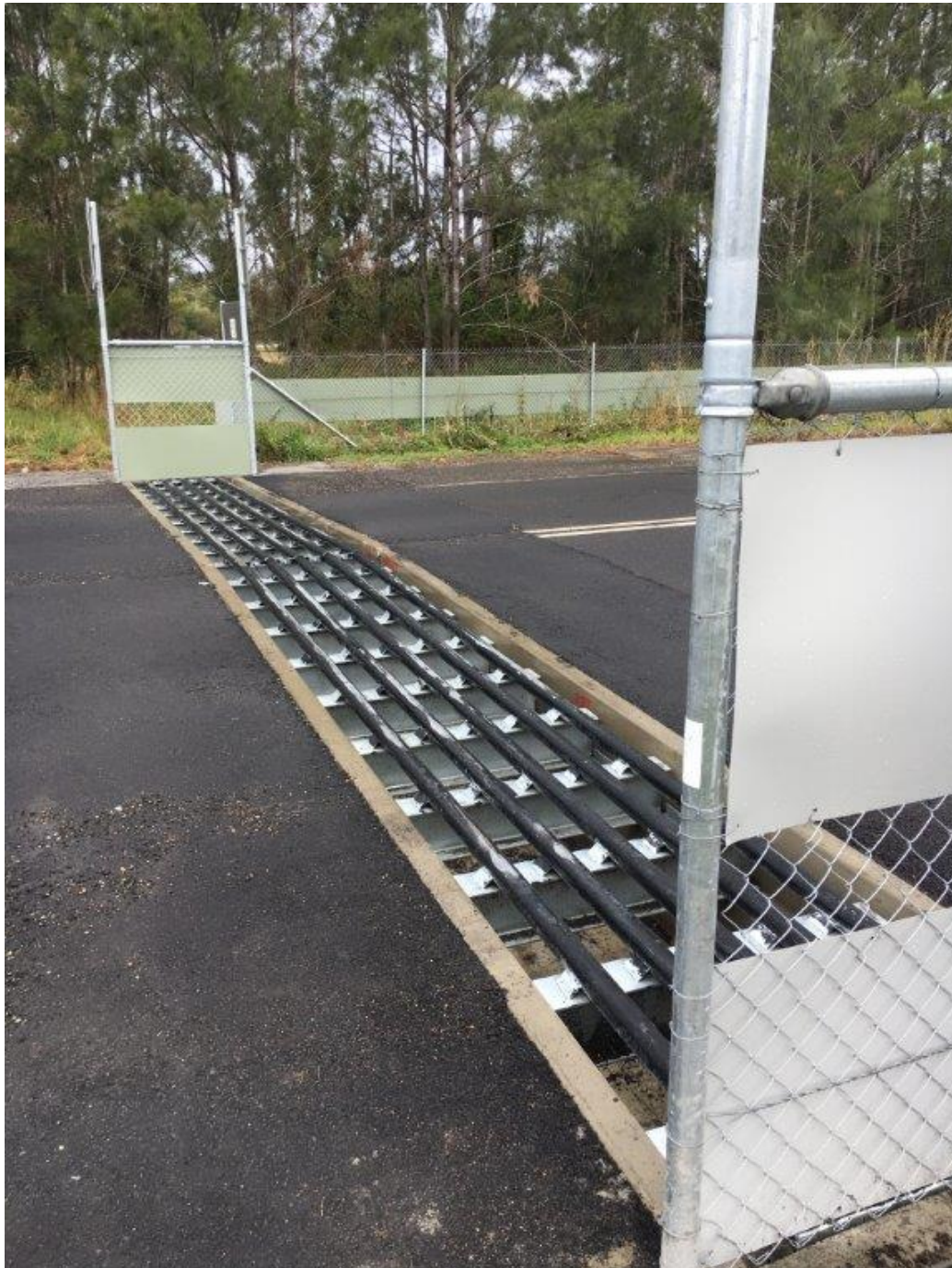
Figure 3: Fence-end – koala-grid interface installation that resulted from the recommendations of Phillips and Fitzgerald (2014).
