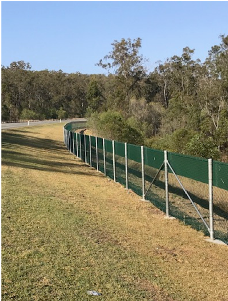
PLATE 1 - example of the proposed amended exclusion fence ( Note : anti-climb panels proposed along bottom of fence)
