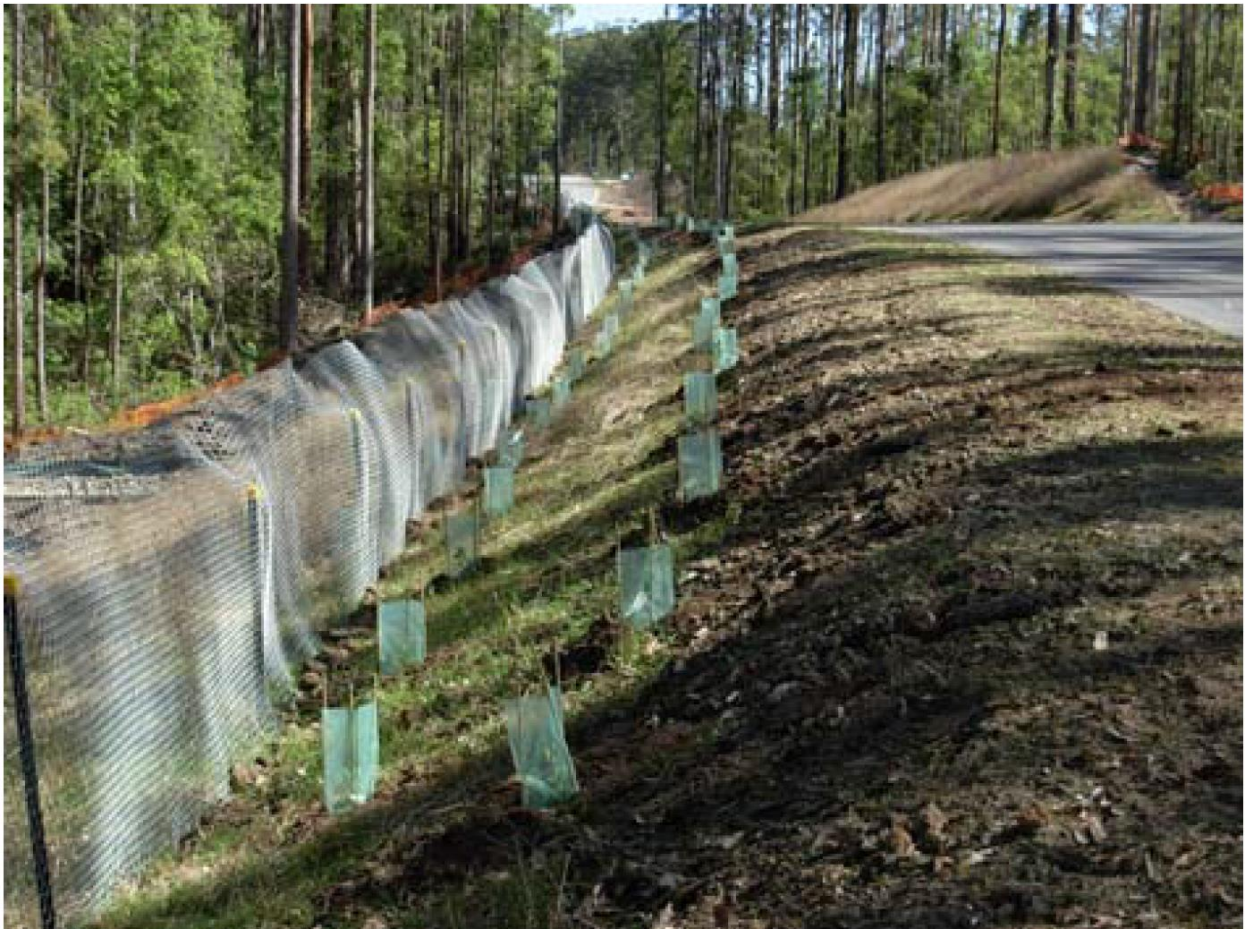
PLATE 1 - EXAMPLE OF TEMPORARY FENCING
