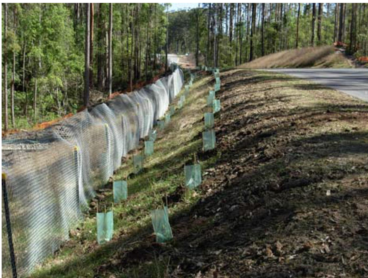
PLATE 1 - EXAMPLE OF TEMPORARY FENCING
