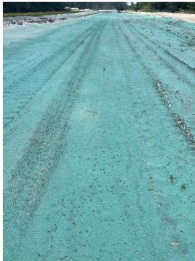
Bed of the eastern Swale polymer application
