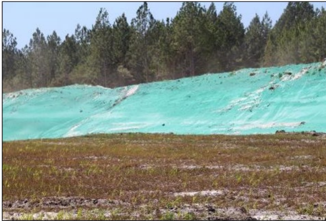
Results of polymer application and grass strike to aide in dust suppression
