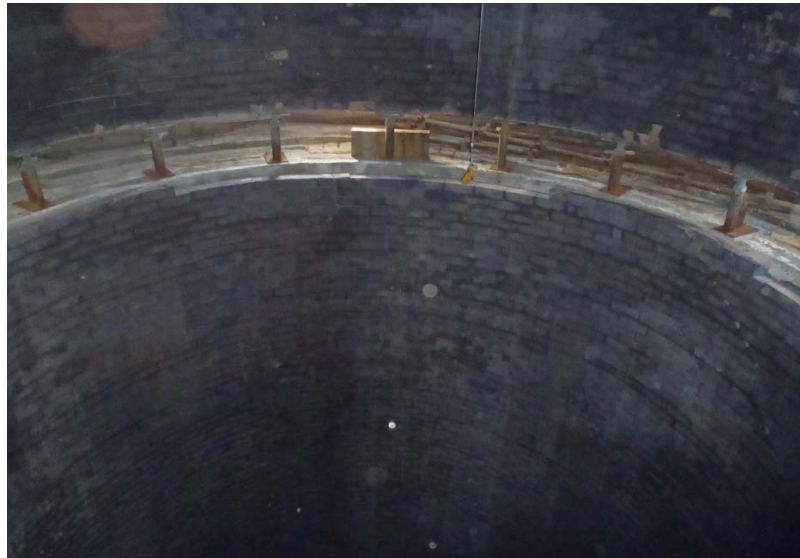
Internal section of stack showing clean bricks
