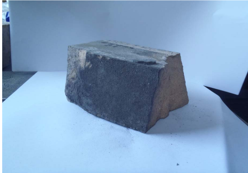
Exposed face of internal stack brick from level 21
