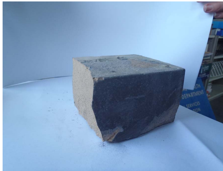
Exposed face of internal stack brick from level 6
