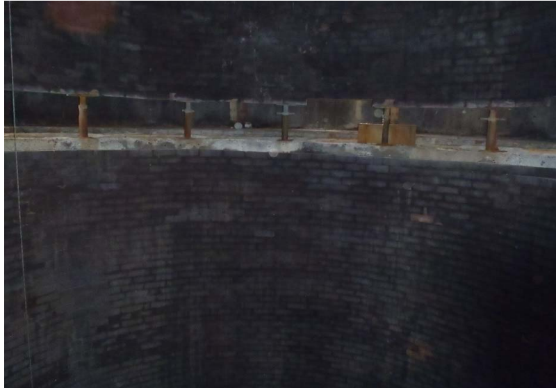
Internal section of stack showing clean bricks and temporary props
