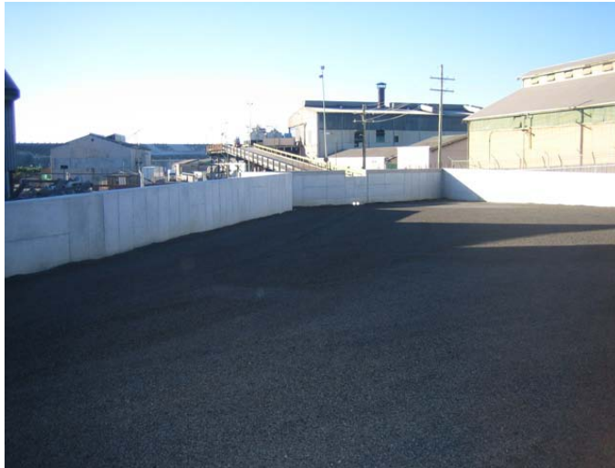
Figure 8 Rehabilitated storage area near 200m stack, showing stormwater management system
