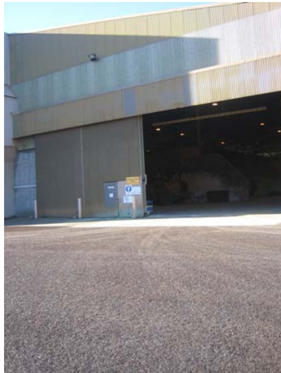
Figure 7 Entrance to Bulk Concentrate Store, showing full capping of surrounding area
