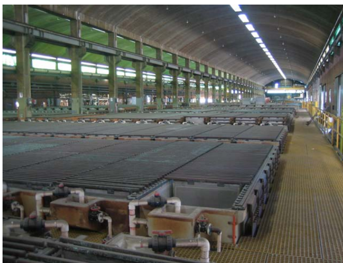
Figure 10 Tankhouse internal view, fully cleaned
