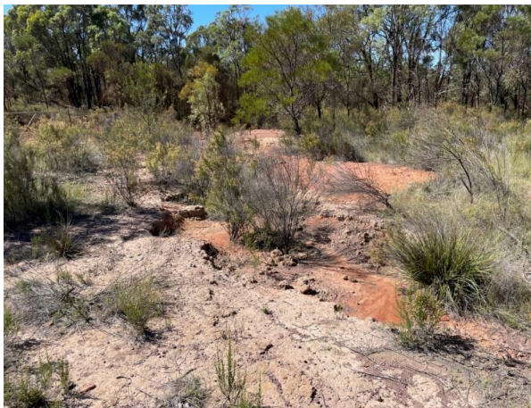
Figure 7: Erosion near Gate 23 identified during 2024
