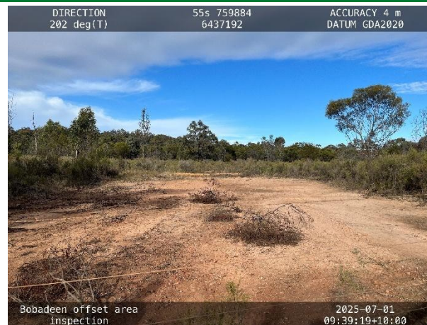
Figure 8: Repaired area of erosion near Gate 23
