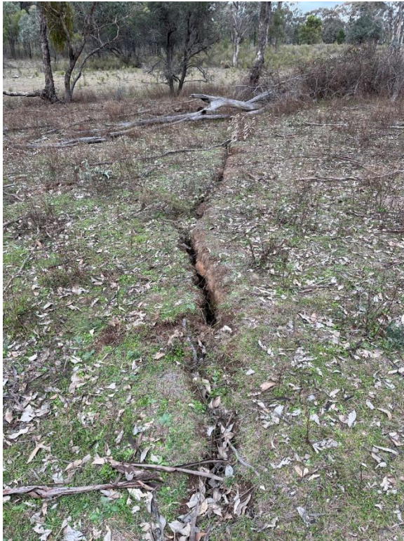
Plate 7: Subsidence crack recorded during Autumn 2025
