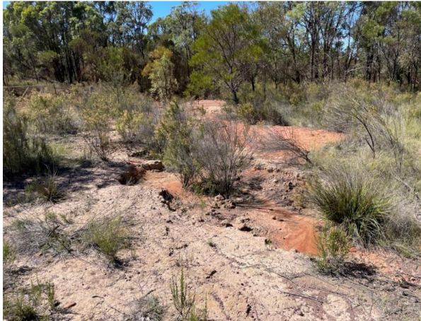
Plate 5: Erosion near Gate 23 identified during 2024
