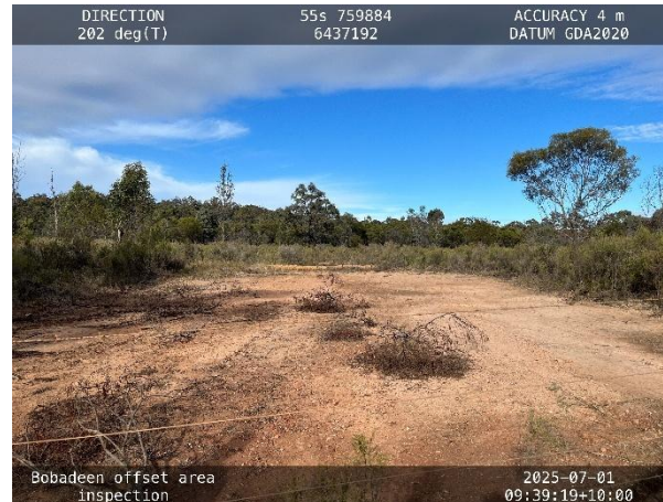
Plate 6: Repaired area of erosion near Gate 23
