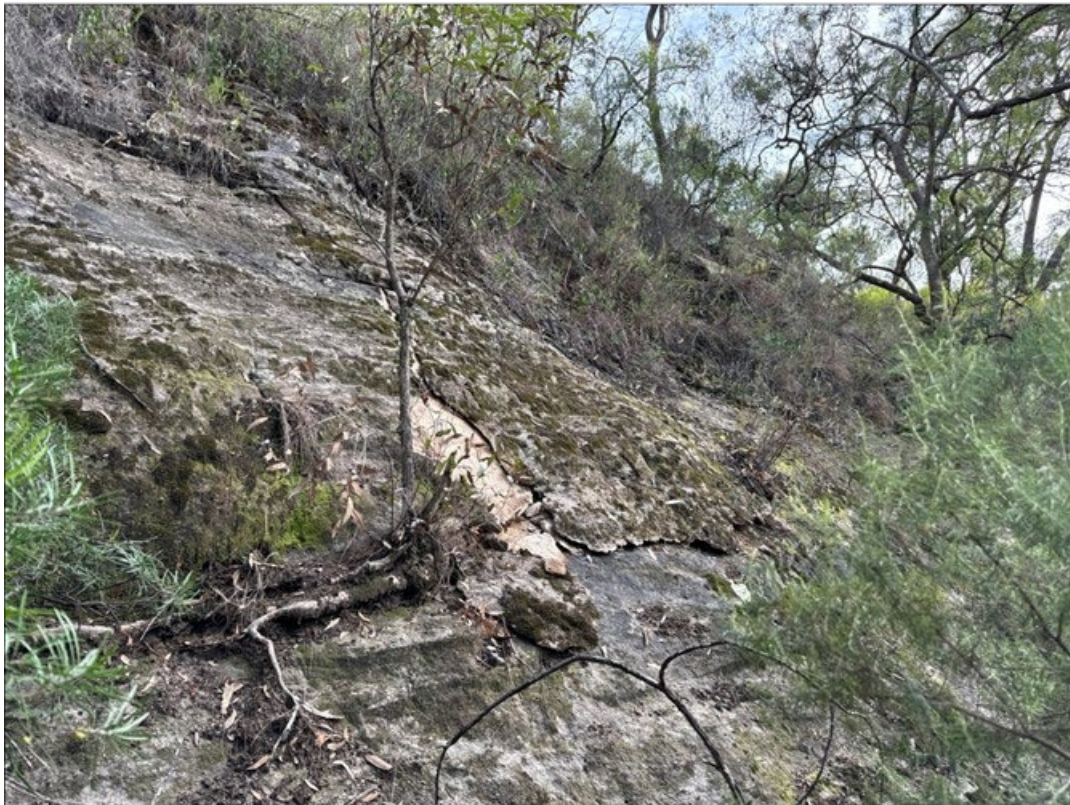
Figure 13: The range of impacts to sandstone outcrop formations above the southern part of Longwall 7 mined in 2024.
