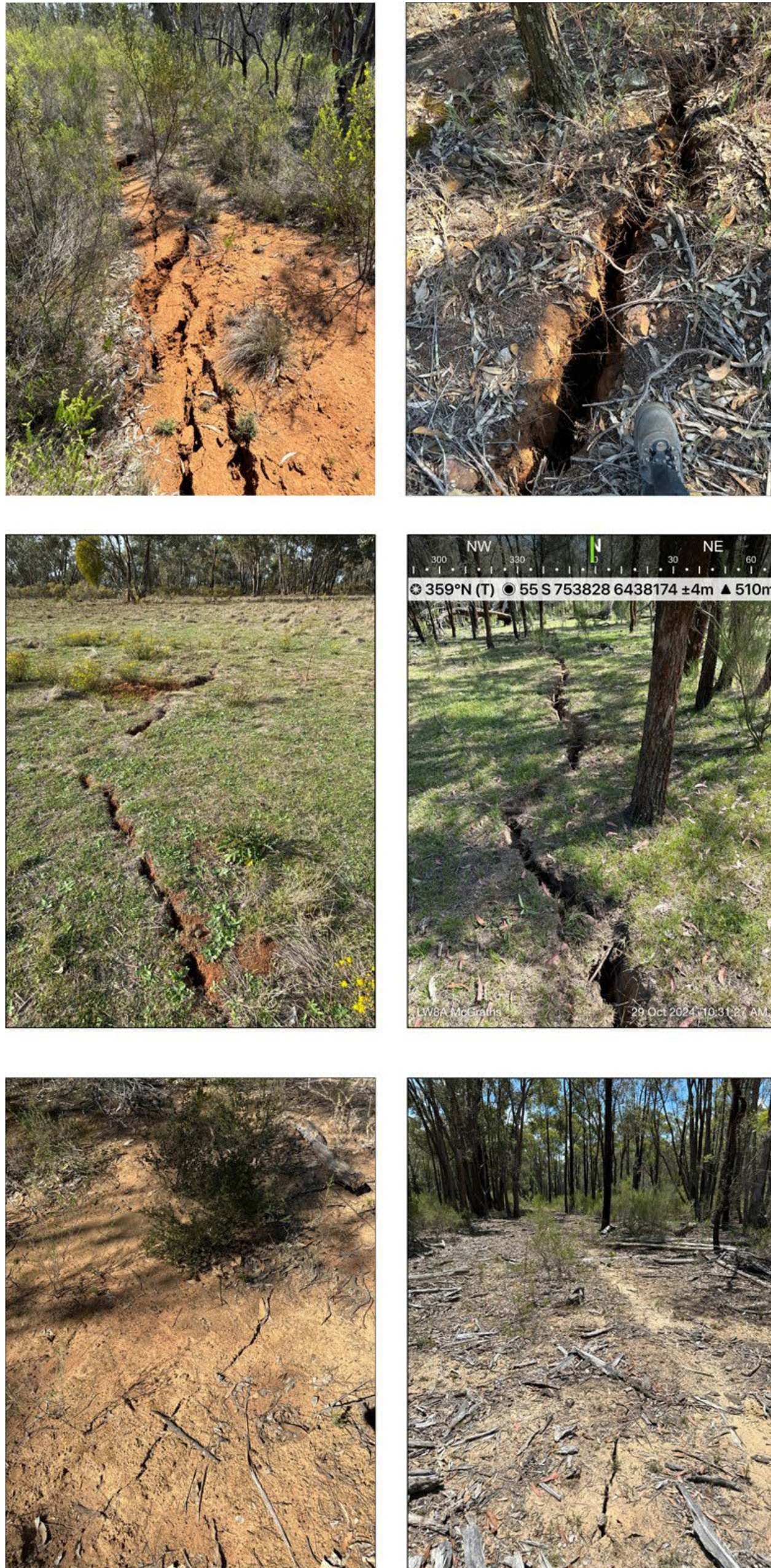
Figure 11: The range of impacts with largest cracks in the shallower areas over the southern part of Longwall 7 and over Longwall 8A and smaller cracks over the central part of Longwall 31.
