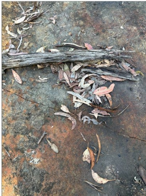
Figure 15: Cracks crossing along the drainage line of Ulan Creek (UCFL4) above Longwall 7 near the Aboriginal heritage grinding grooves site (Ulan ID#1210).
