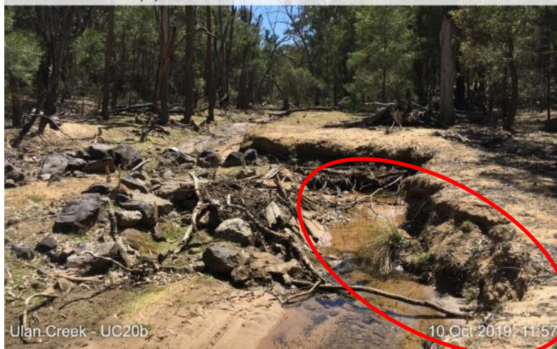
Continuation of material loss from LHB in 2019 and slumping of the creek bank.
