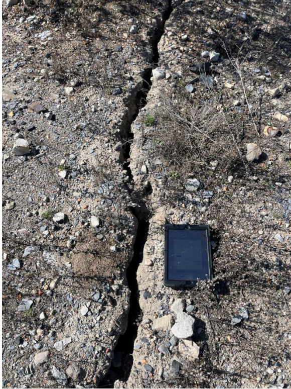
Plate 1: Landform settlement cracking in Polygon 5
