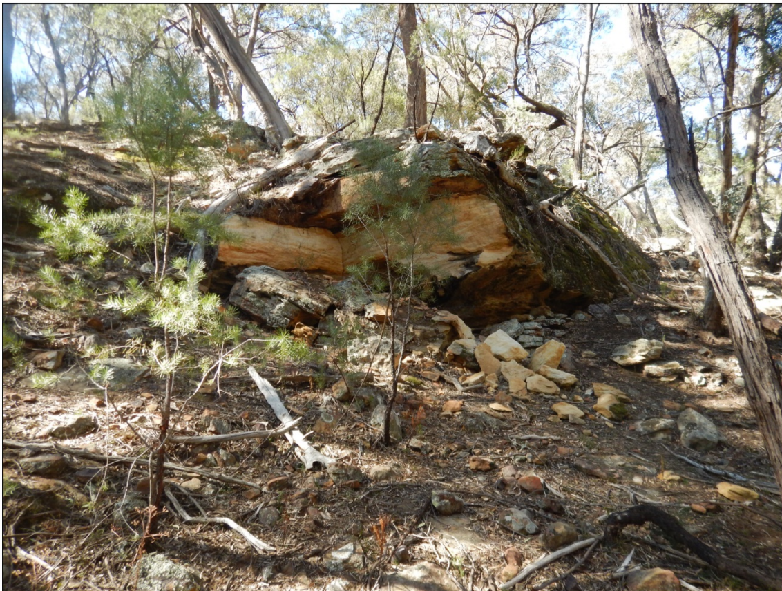
Figure 3b: Top photo shows sandstone outcrop formation with no perceptible impacts and bottom photo shows another section of the same formation with rock fall at Aboriginal heritage site Ulan ID#479 (MC45A) above Longwall W3.
