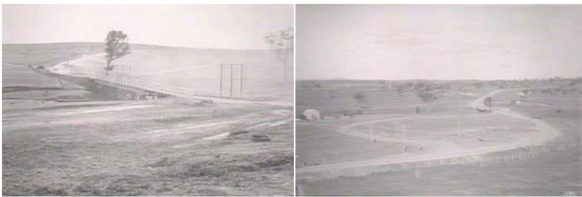
Figure 2. Glennies Creek New England Highway crossing. Photographs dated 1936. Left is looking west from Camberwell and right is looking east. Photographs from State Library NSW (cannot be copied or reproduced).
