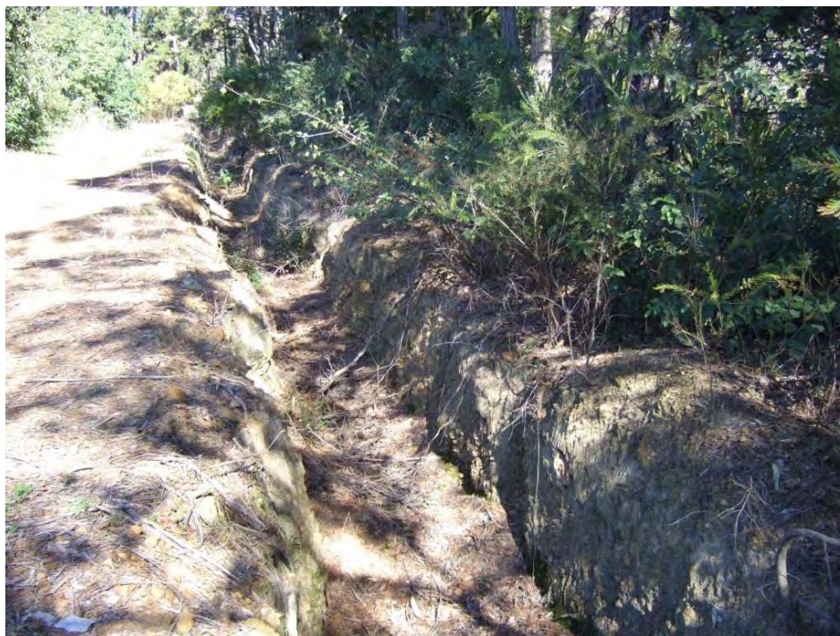
Plate 5: SU3 Access Road – view to south of showing farm access road and excavated drainage channel
