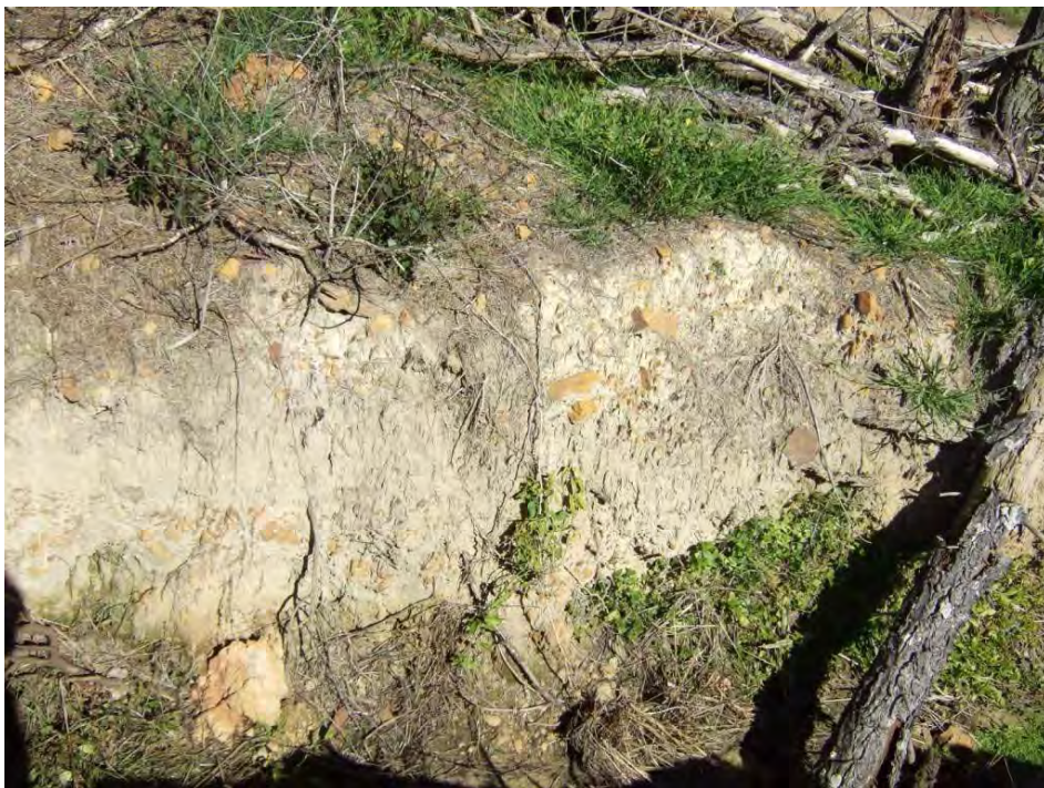
Plate 16: SU5 Excavated Drainage Channel – view to south east showing soil profile with friable limonitic sandstone pebbles and cobbles
