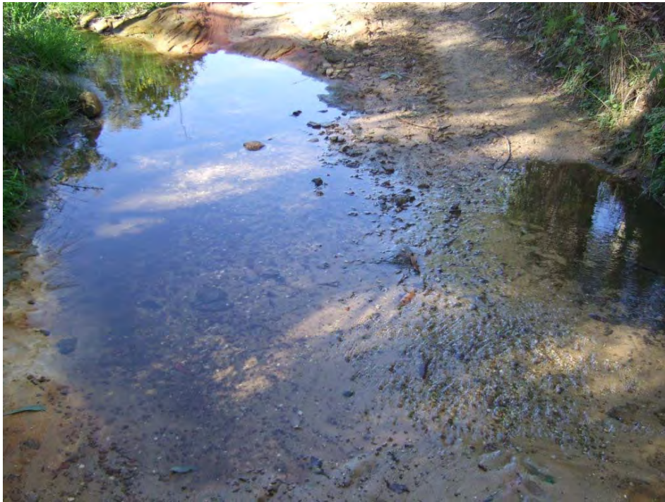
Plate 11: SU4 Creek Crossing – view to south east showing access road to dam and diverted creek channel
