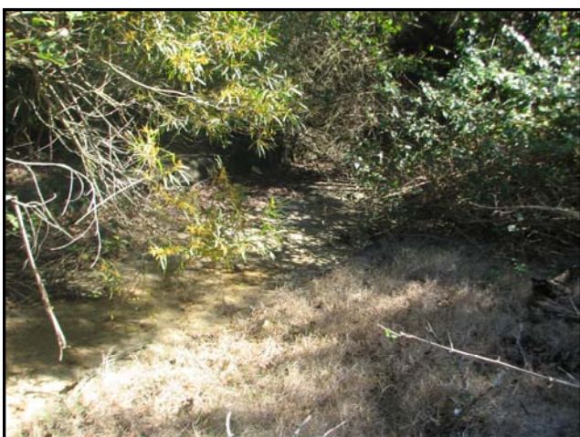
'Point 1' outlet – concrete lined channel
