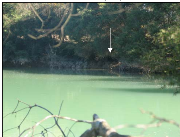
'Point 1' inlet and pump dam
