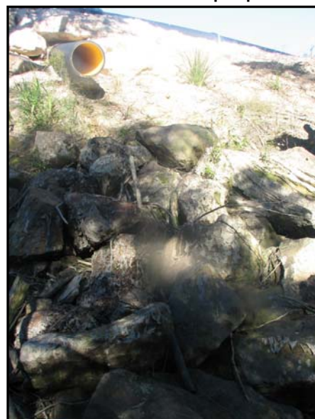
'Point 2' outlet – rip rap
