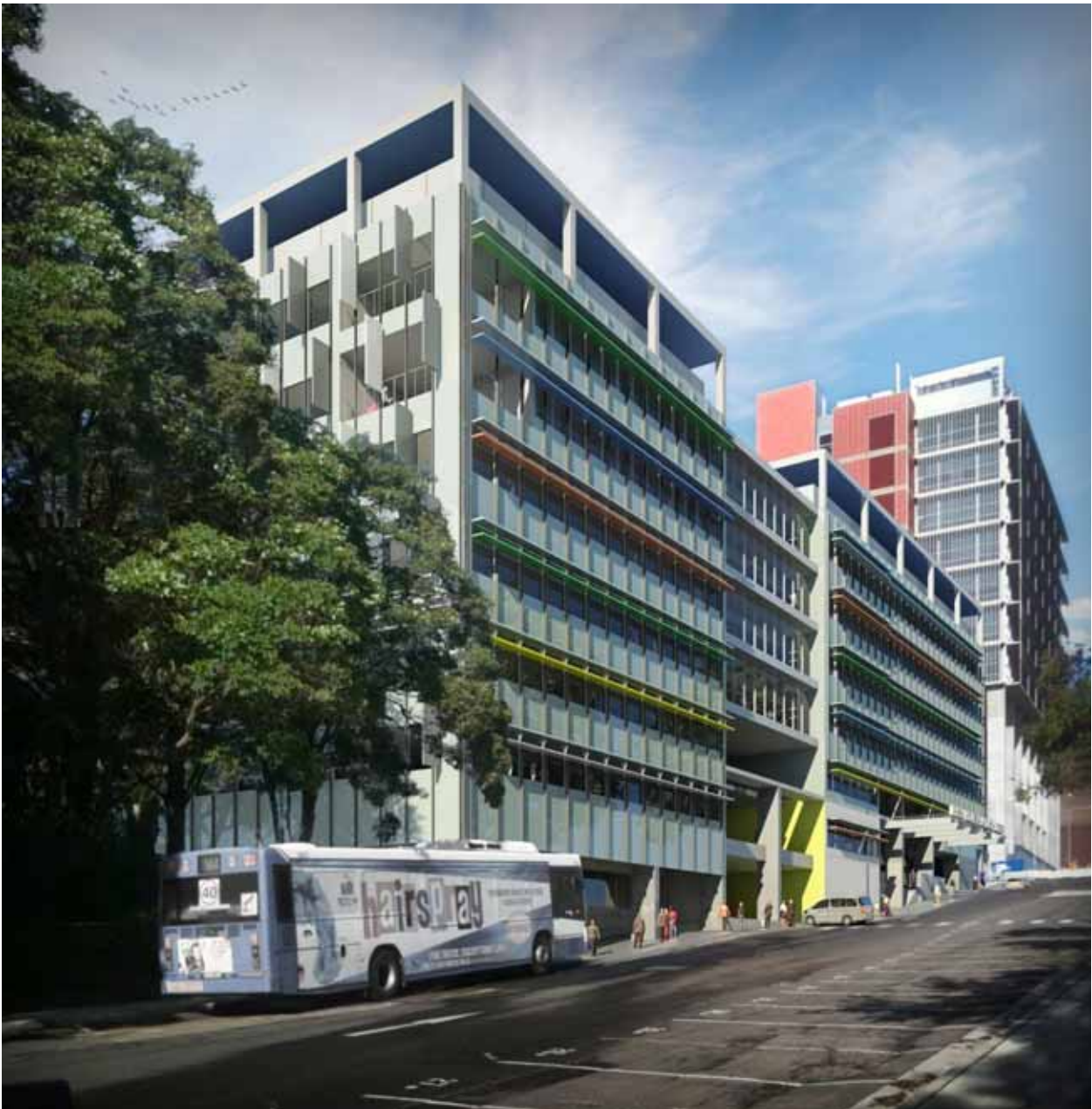
FIGURE 7 – INDICATIVE STREETSCAPE VIEW ALONG THE SOUTHERN SIDE OF WESTBOURNE STREET LOOKING WEST - HASSELL
