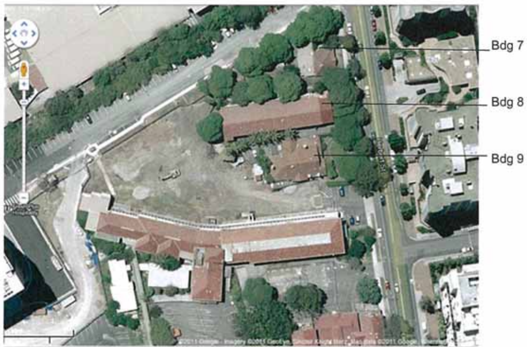
Figure 1.2 Aerial photo of site during construction of temporary car park—note removal of trees. (Source: Google maps).
