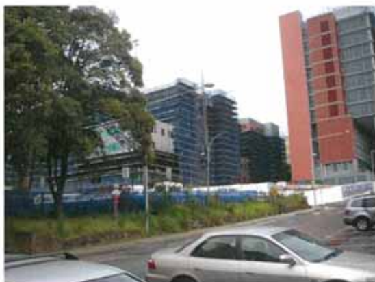
Figure 2.1 Looking west along Westbourne Street to the development site. The Kolling (Research) building is on the right hand side, and the Acute Services building is in the background.
