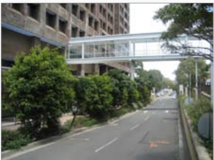
Pedestrian overpass Westbourne Street
