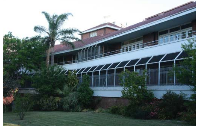
Figure 3-2 Northern facade of the building's original west wing, shows details of the enclosed verandah
