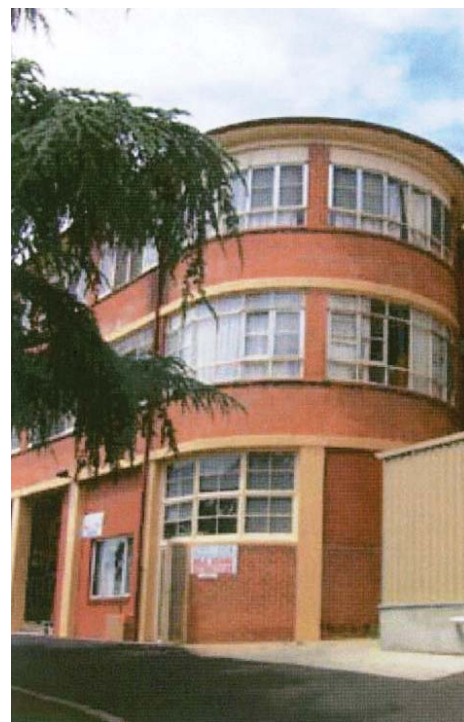
Figure 4-5 Maternity Wing Bathurst District Hospital
