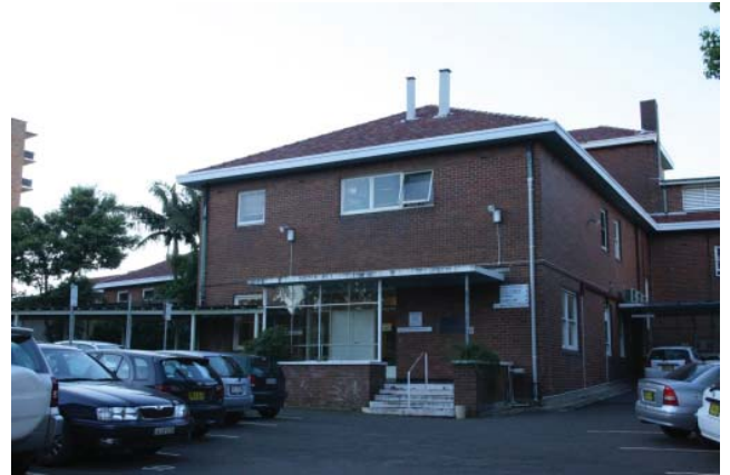
Figure 3-6 Rear (south) elevation of the central building element
