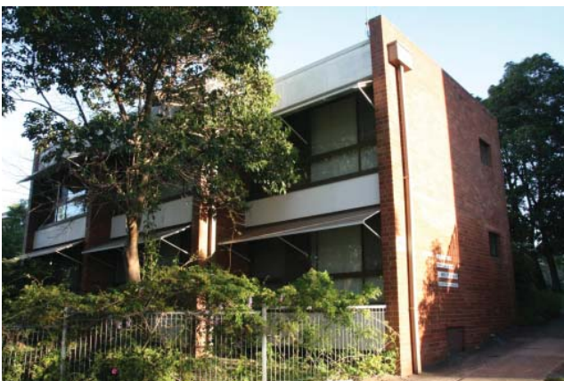
Figure 3-9 Two storey 1980s western addition
