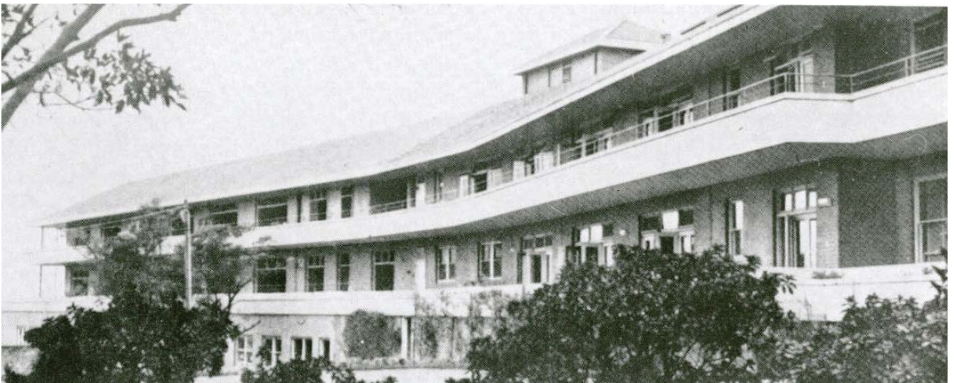
Figure 2-4 Photograph of Building 10, looking south east
