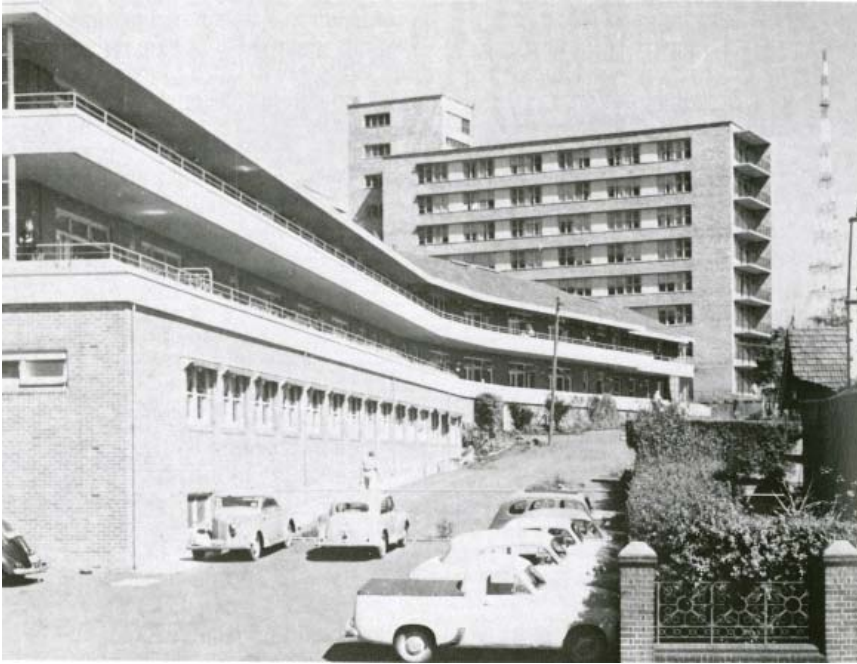
Figure 2-3 1956 photograph of the extended Building 10, looking west from Herbert Street
