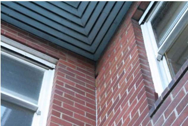
Figure 3-7 Shows detail of the vented eaves of the western wing of the southern facade
