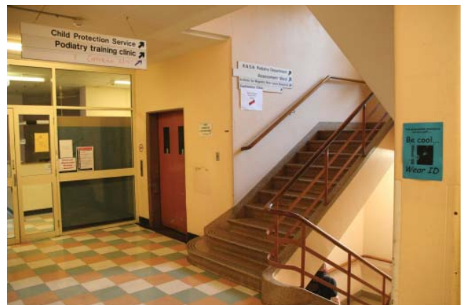
Figure 3-10 View of the central stair well with its terrazzo stairs
