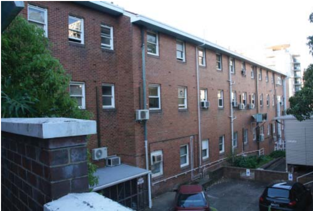
Figure 3-5 Shows the rear (south) elevation of the building's east wing
