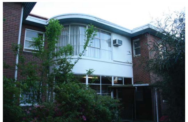
Figure 3-3 Curved entrance at rear of the building.
