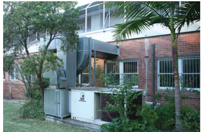
Figure 3-8 View of the north elevation of the east wing
