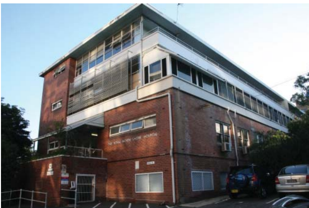
Figure 3-1 View of Building 10 from Herbert Street, showing the east and north elevations
